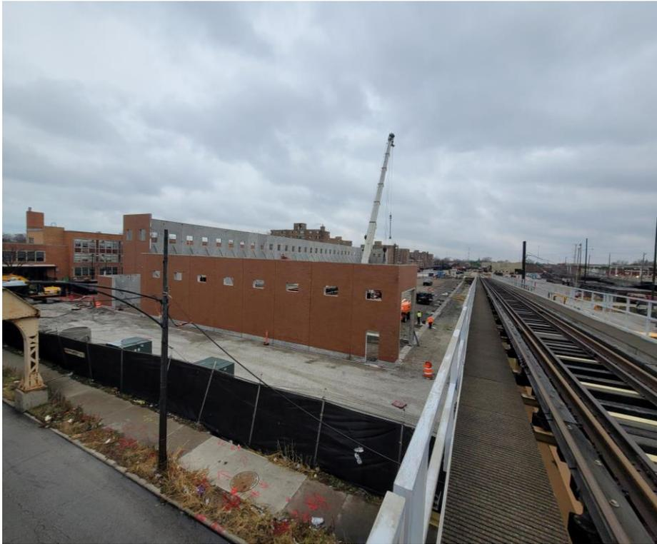
**New Horizon – Precast Panel Erection – North Wall**
