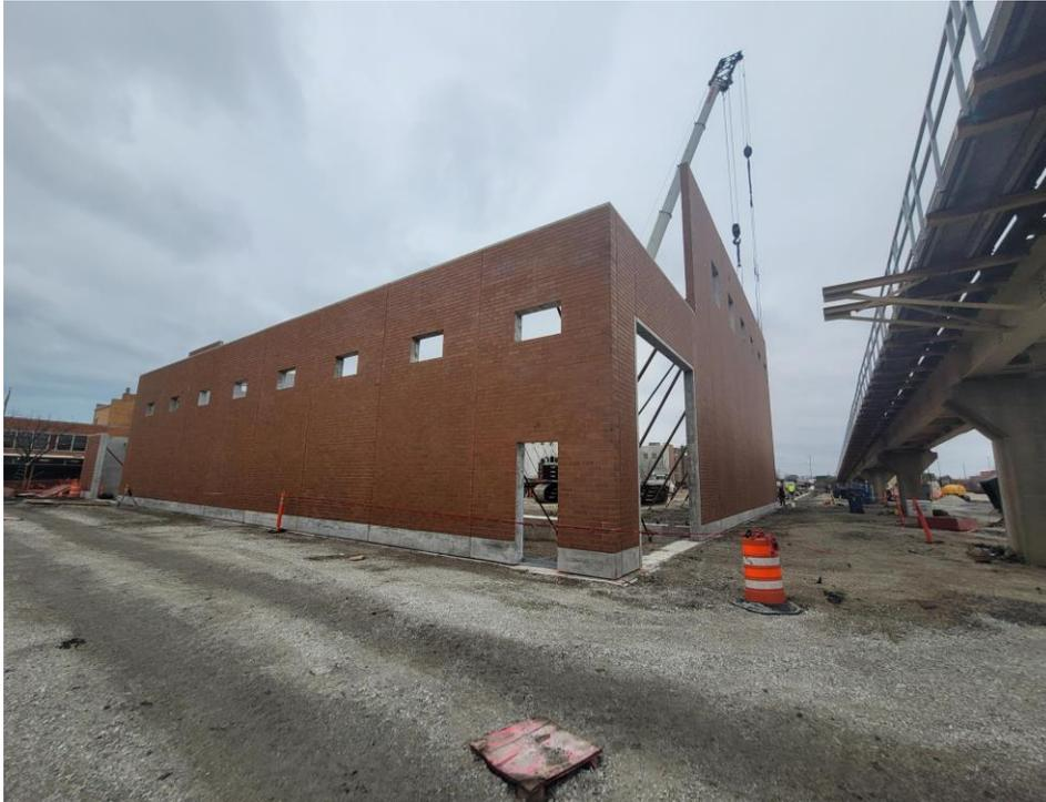
**New Horizon – Precast Panel Erection – Loading Dock**
