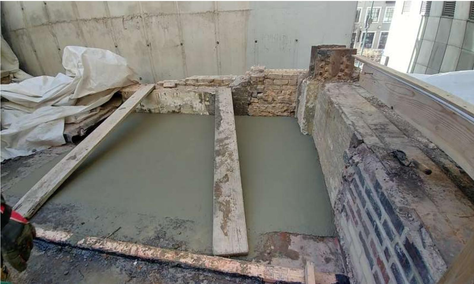
Concrete Roof Pour at East Lake Substation
