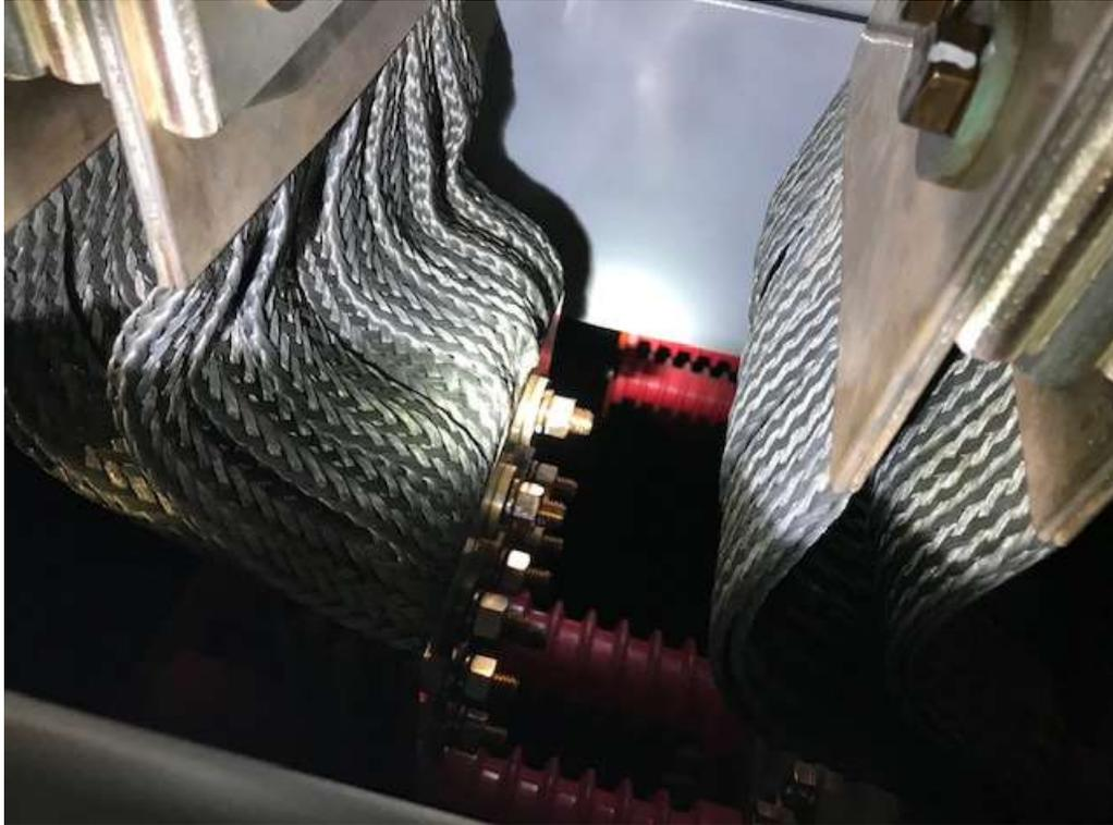
Rectifier Transformer Line Up #2 Connections Installed
