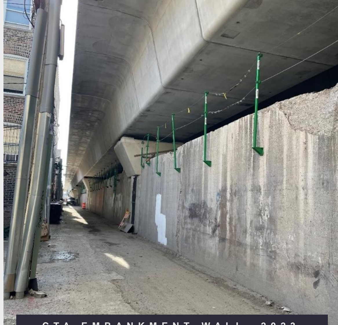
CTA EMBANKMENT WALL, 2023
