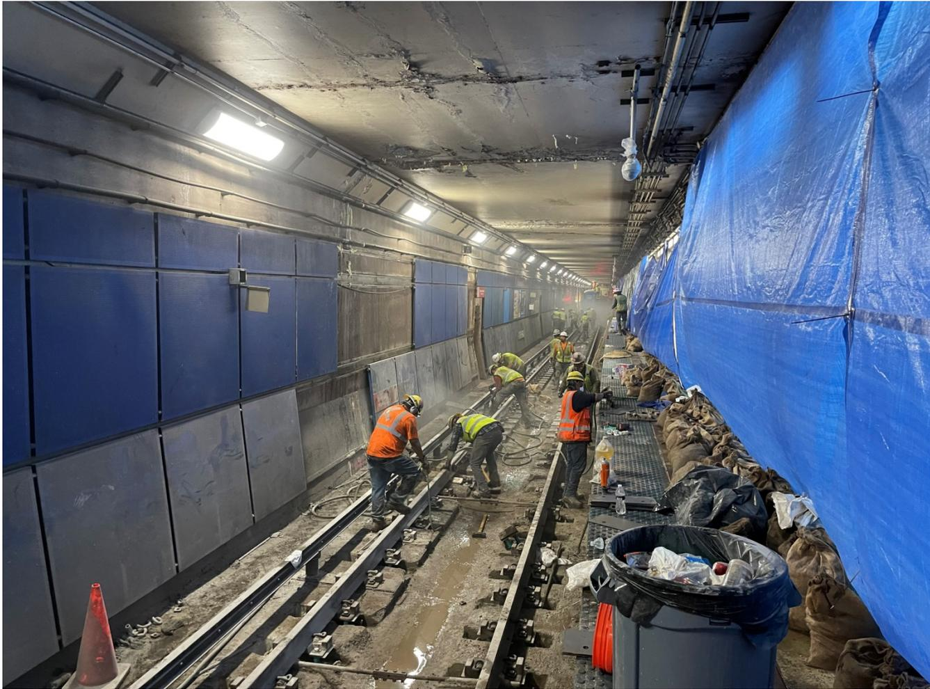
**Pouring and finishing of new concrete track ties**
