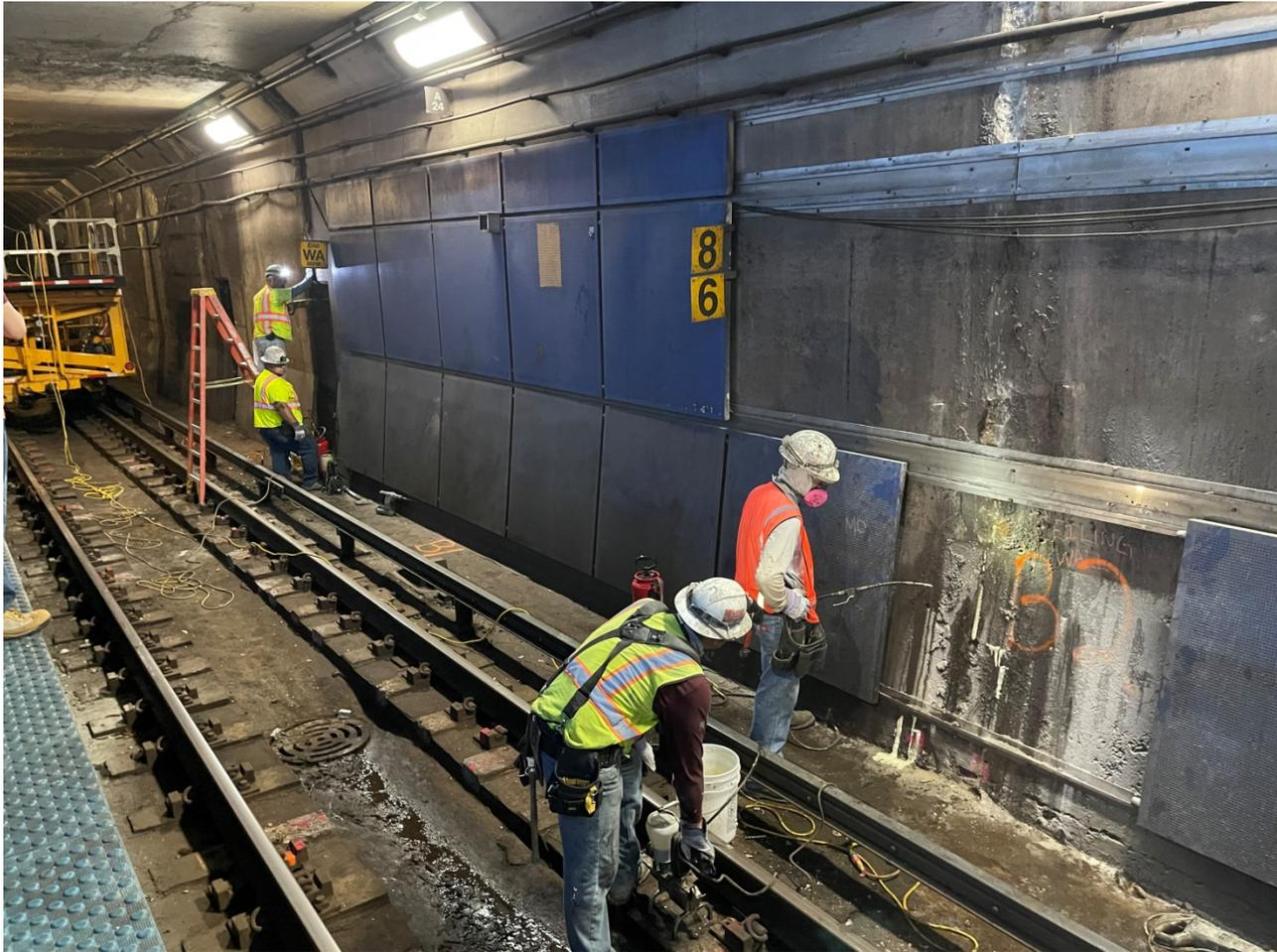
**Removal of existing acoustic sound panels by CTA's Facility Maintenance crews**
