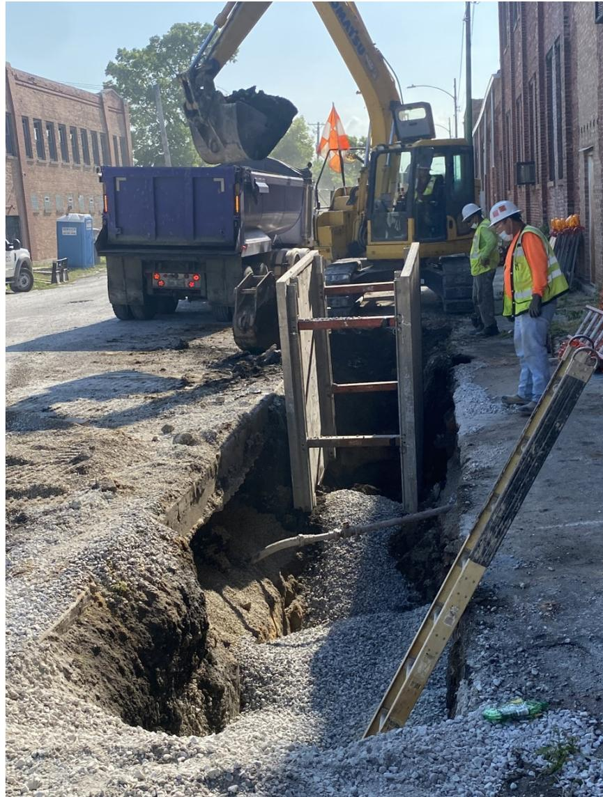
**Demolition and installation of trench shoring for Sewer Replacement**
