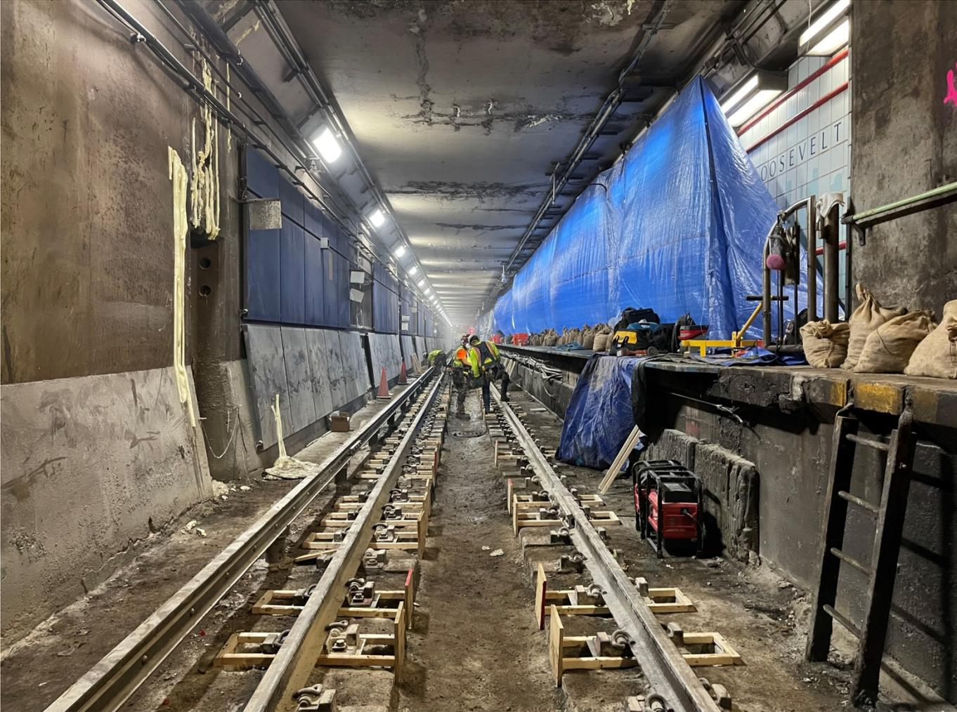
**Installation of concrete forms for the new concrete ties.**
