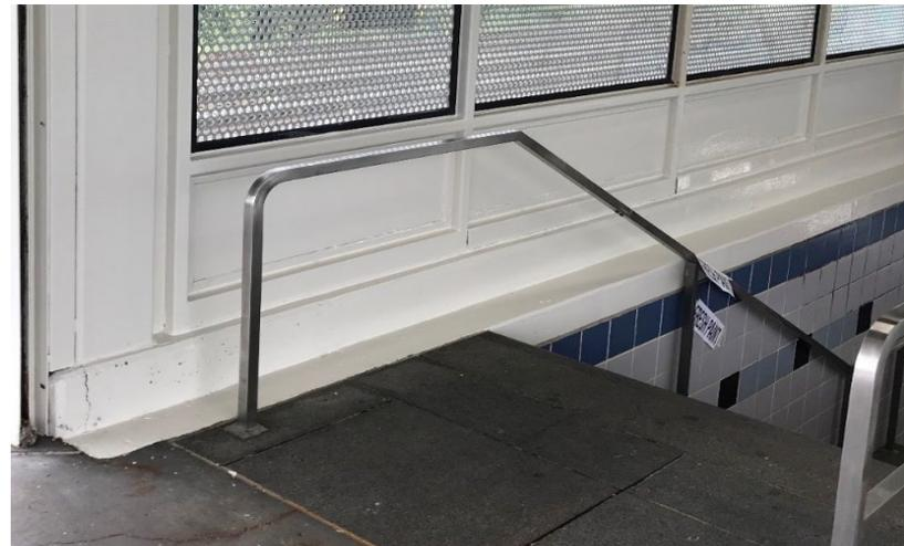
**Kedzie (Orange Line) Repaired rusted sections of stairway storefront along with fresh coats of paint and rust inhibitor**
