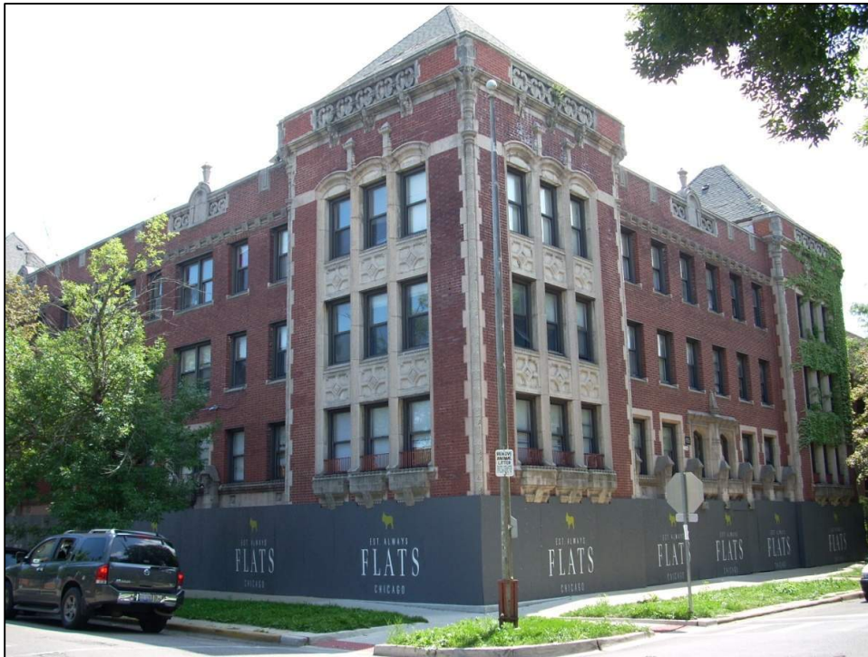
Figure 5-8: North and West Facades of 4875 N. Magnolia Avenue Apartment Building
