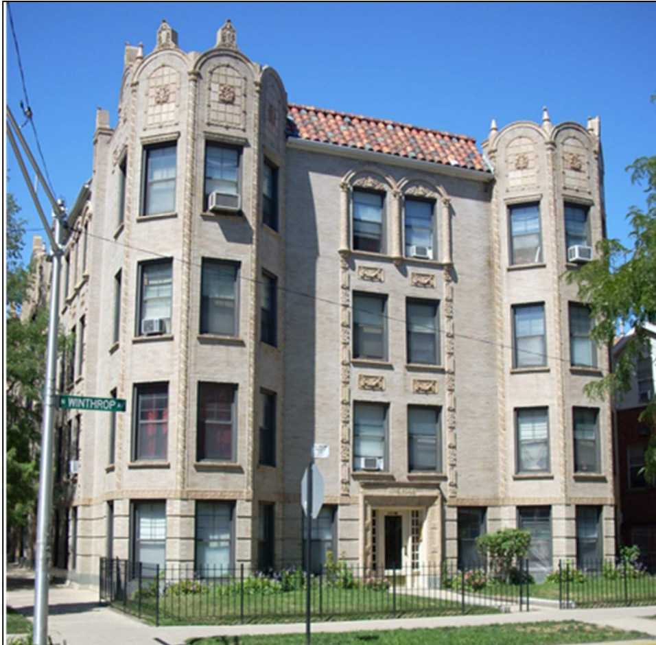
Figure 5-12: East Facade of the Rose, a Spanish Revival Apartment Building
