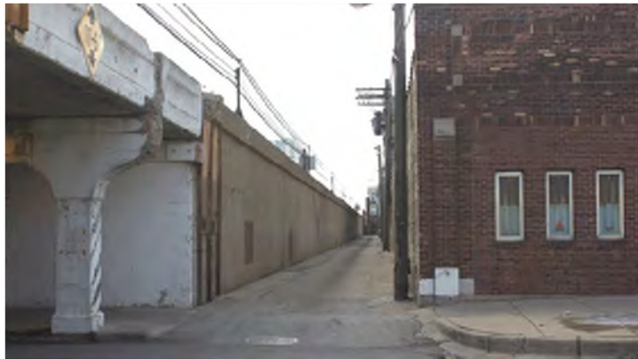
Concrete retaining wall and viaduct
