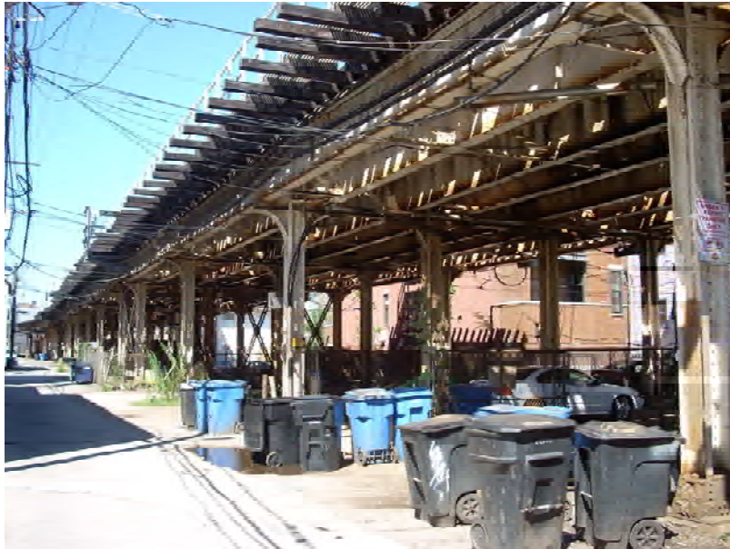
Steel structure near Belmont Station
