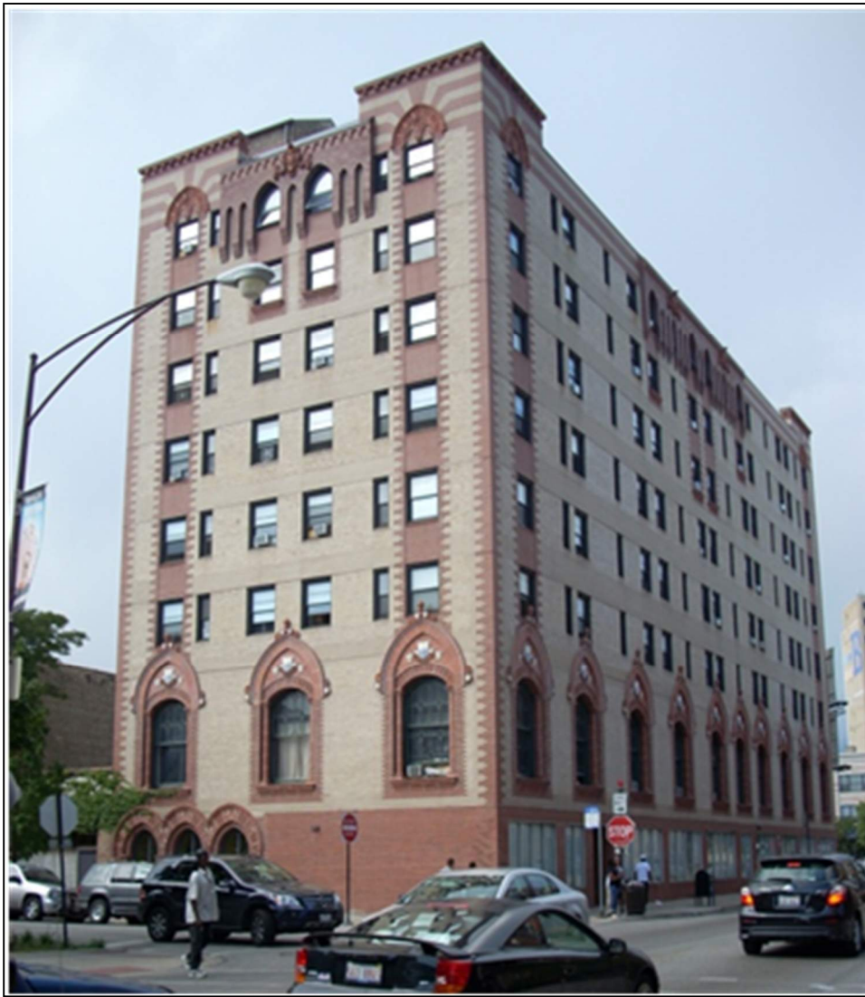
Figure 5-6: North and East Facades of the Wilton Hotel Apartment Building
