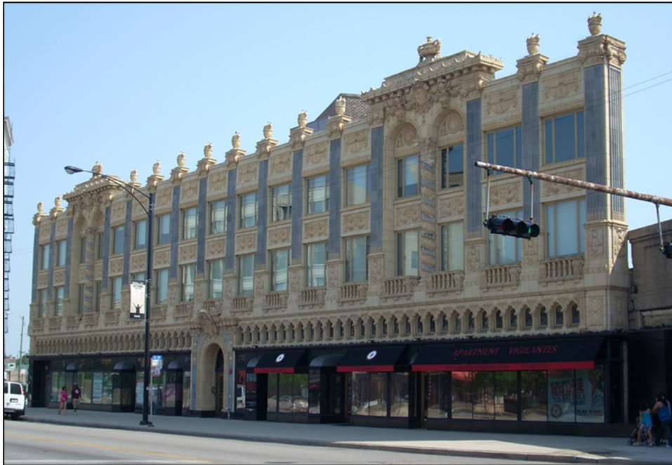
Figure 5-1: West Facade of the Uptown Broadway Building
