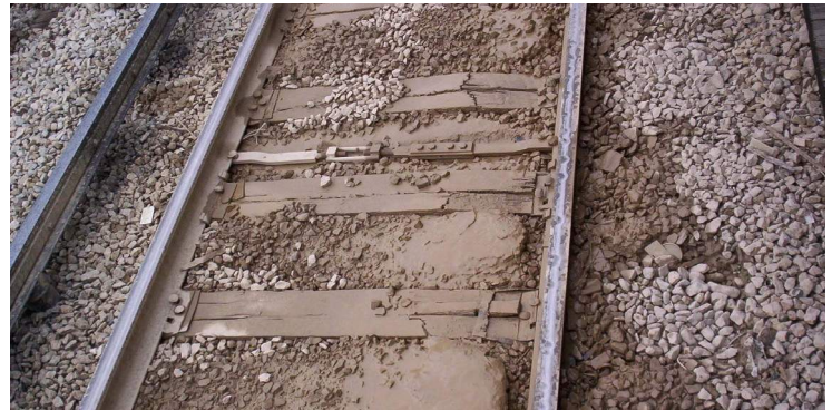
Deteriorating timber ties
