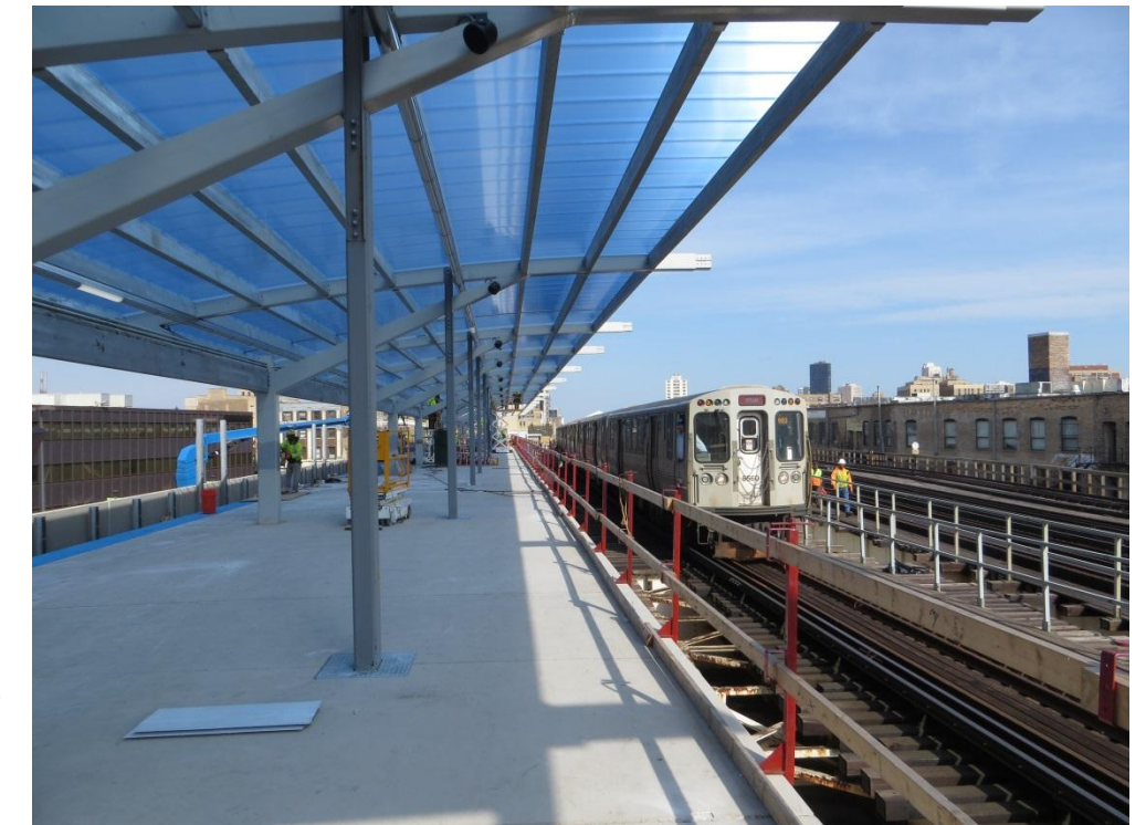
(Right) New Wilson platform under construction
