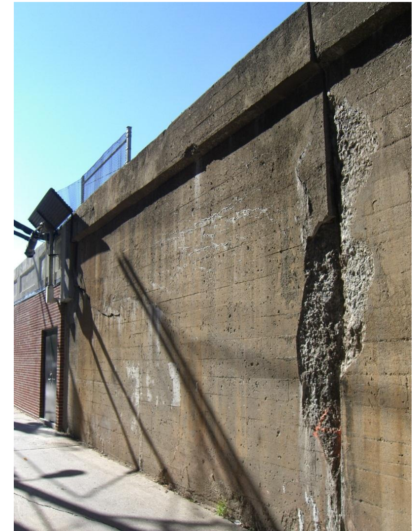
Deteriorating Embankment
