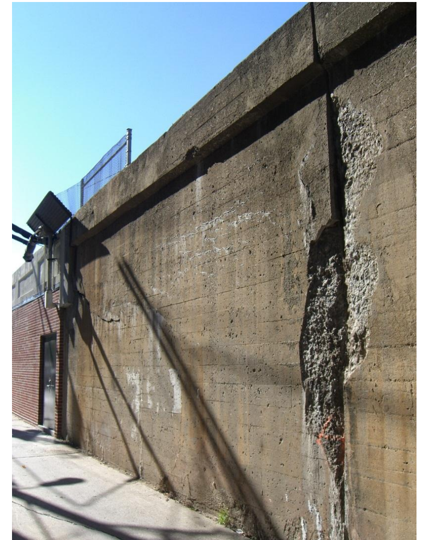
Deteriorating Embankment
