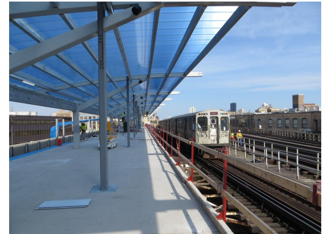
(Above right) Aerial view of new west island platform as part of historic Wilson Station Reconstruction Project
