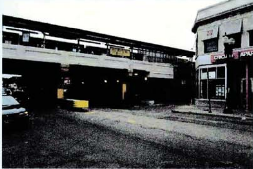
Existing Viaduct at Bryn Mawr Station
