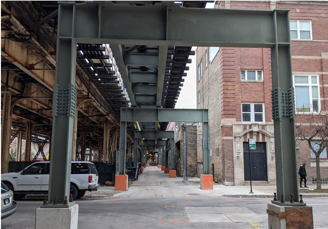
New temporary track over alley west of Red & Purple Line tracks, facing south.
