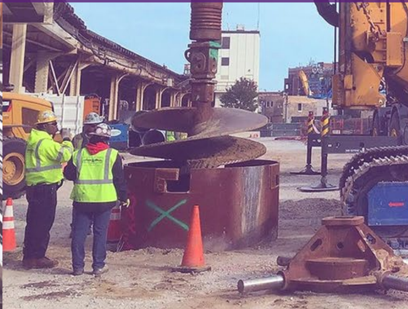
Drill new track foundations
