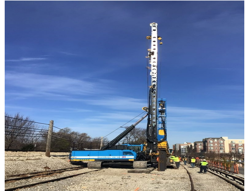
RPM sheet pile driving testing on the Purple Line with noise monitoring, November 2020
