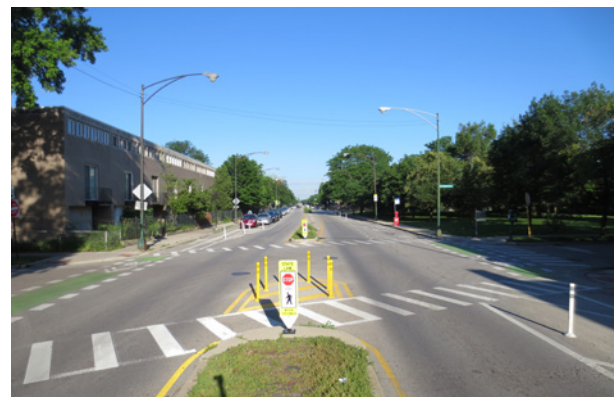
Figure 95. CDOT 55th Street mid-block crossing (CDOT)
