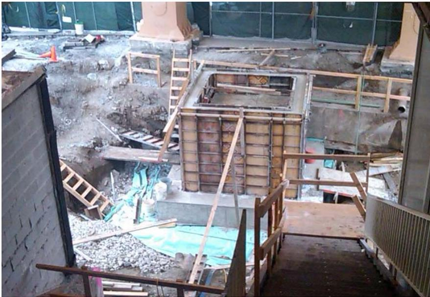
**Excavation and forming of elevator foundation**
