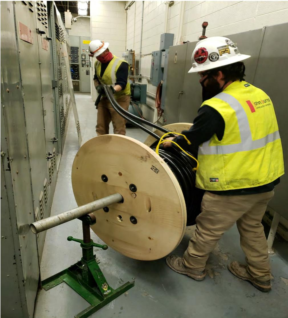
**Setting Up for Cable Pulling for Transformer #3 at Edmunds Substation**
