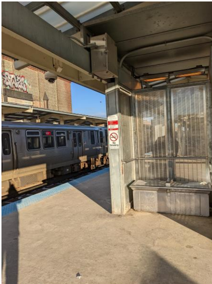
Seating at Belmont station.
