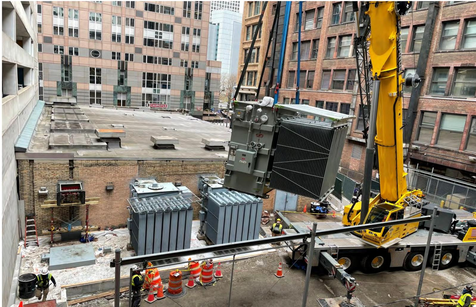
**Hoisting Transformer 1 at Franklin Substation**
