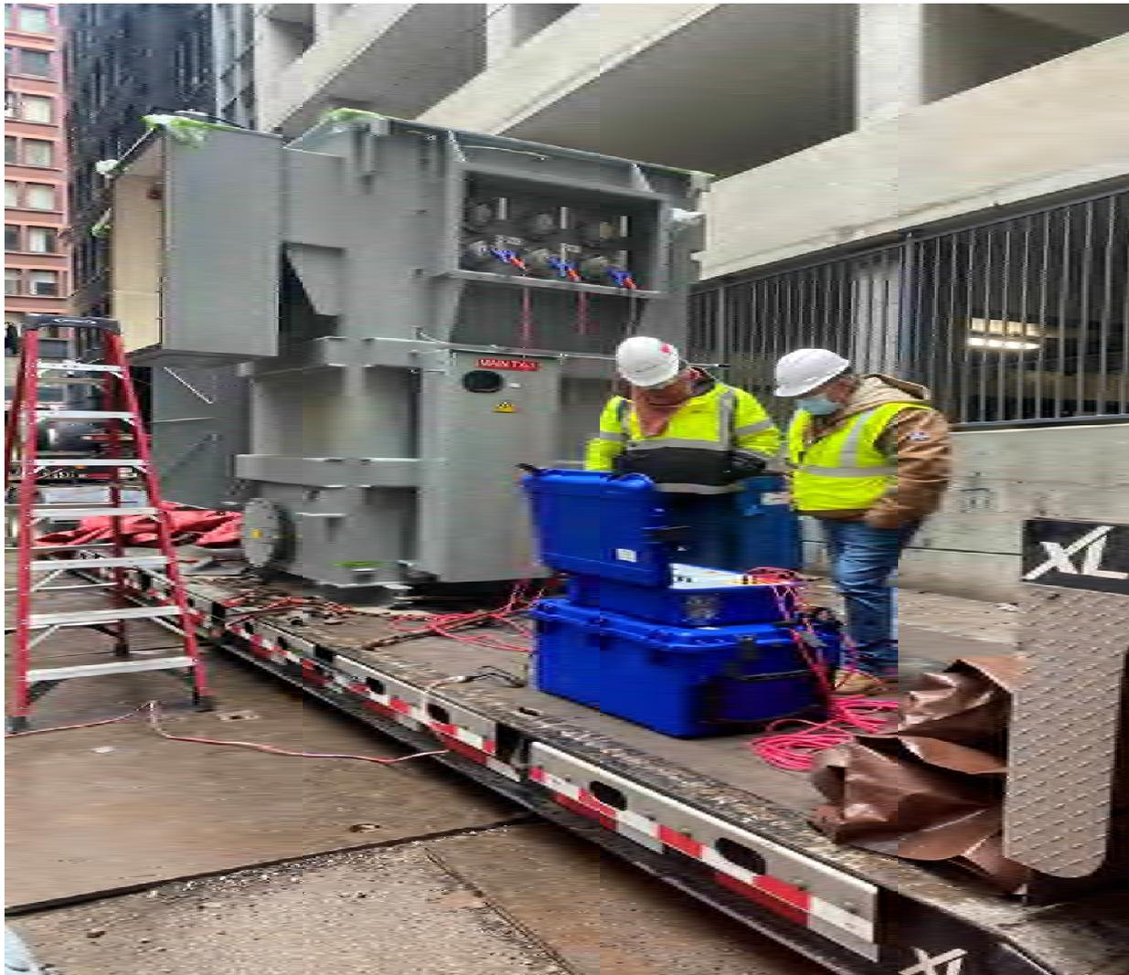
**Field Testing New Transformer 1 on Flatbed at Franklin Substation**
