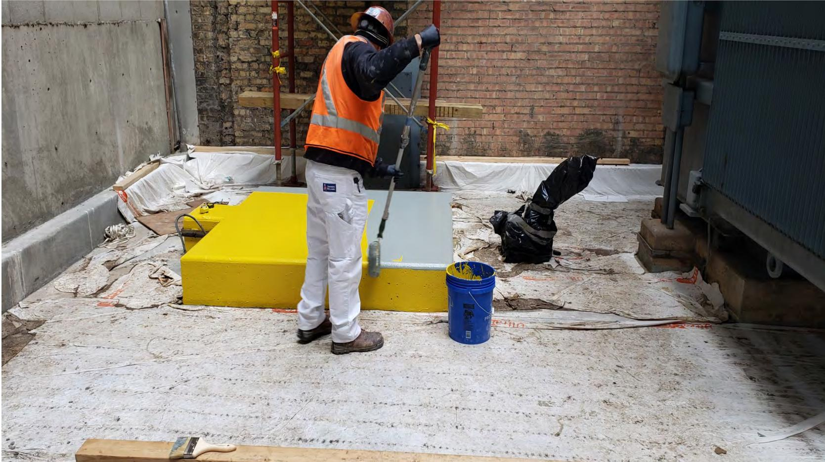
**Applying Epoxy Coat over Concrete Pad 1 for Transformer 1 at Franklin Substation**
