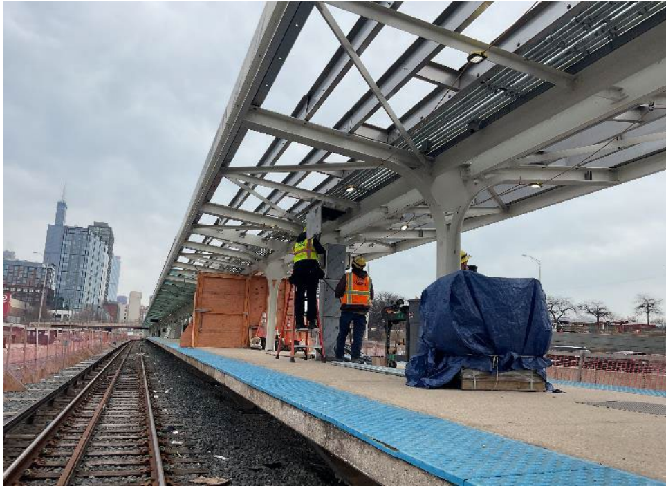
Platform Purlins Installation Near Loomis
