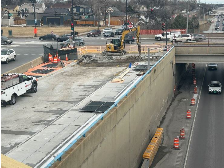
Demolition of Pavement at Harlem
