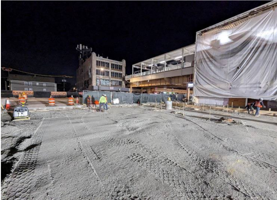
South BTA – Base Course Compactions
