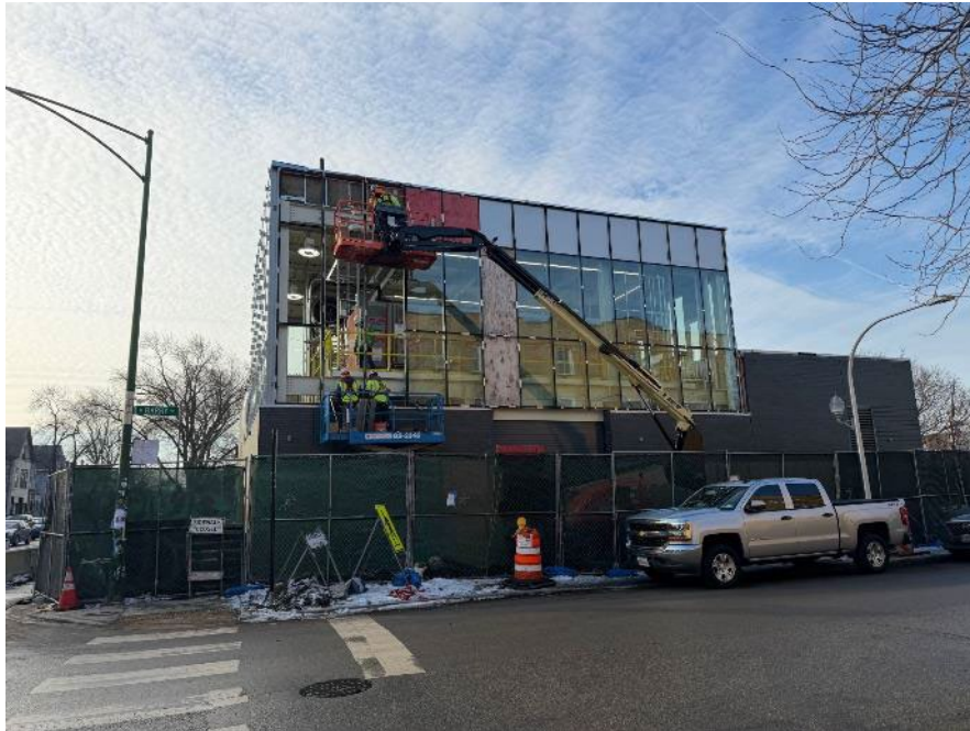
Barry Curtain Wall Installation
