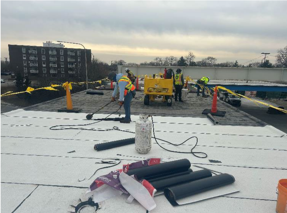
Roofing Membrane at Bus Canopy
