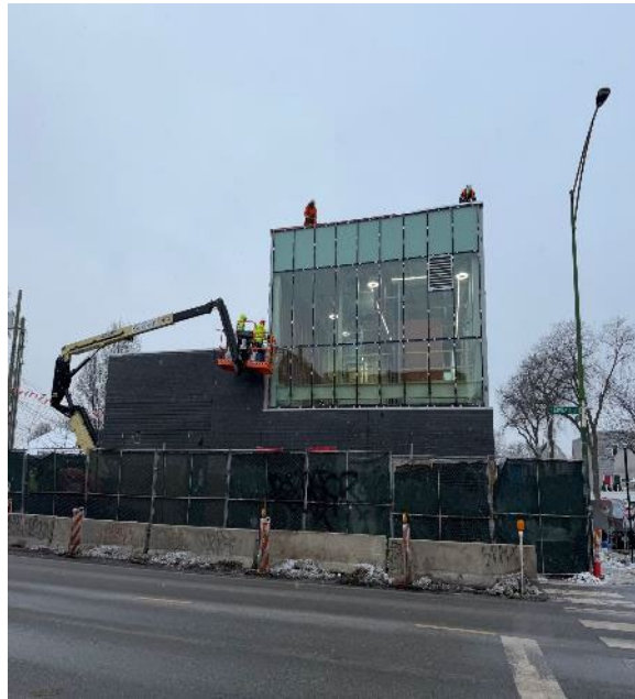
Barry Curtain Wall Installation
