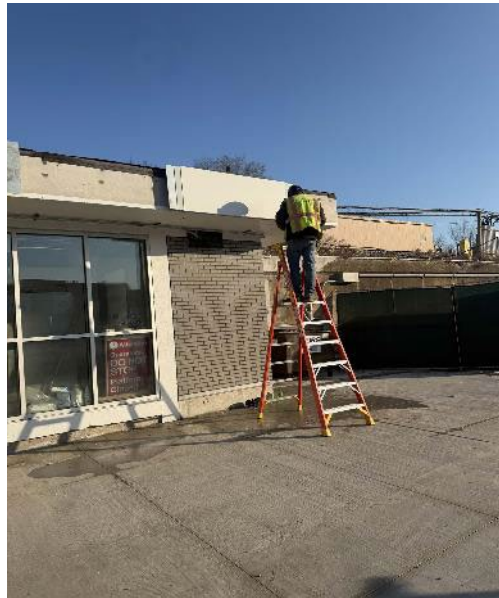
Completing Glazed Masonry and In-Progress Fascia Installation
