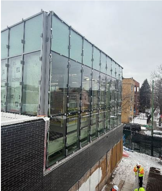
Barry Curtain Wall Installation
