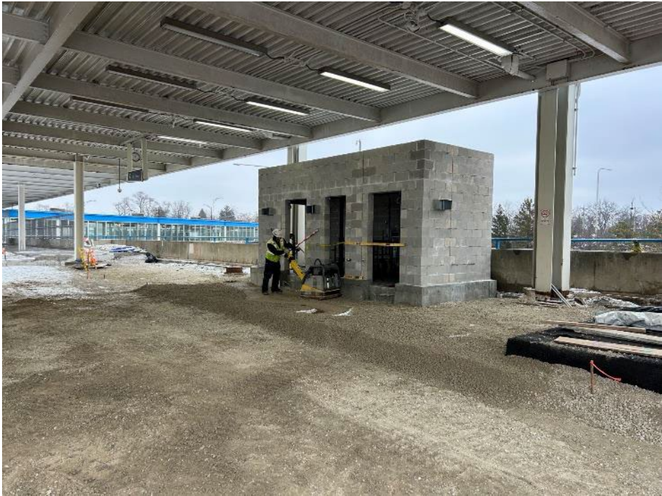
Final Grading Around Bus Washroom
