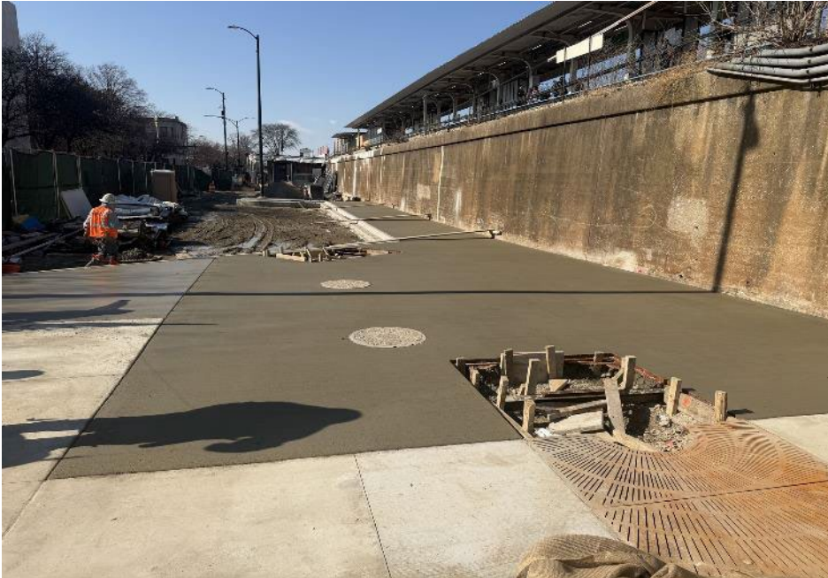
Pouring Concrete Curbs and Flatwork
