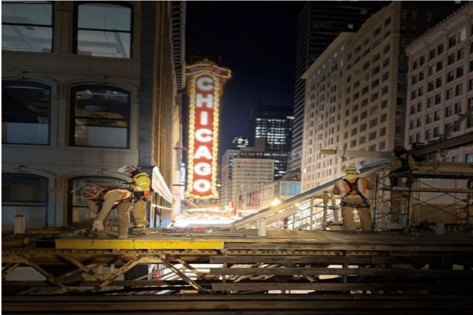
Elevated Platform Demolition
