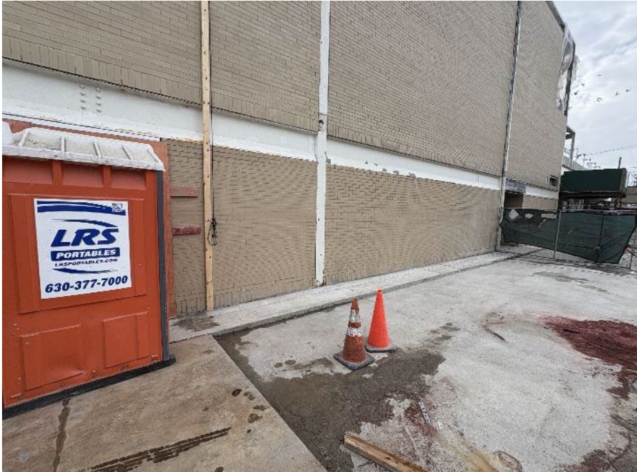
North Facade - Completed Masonry
