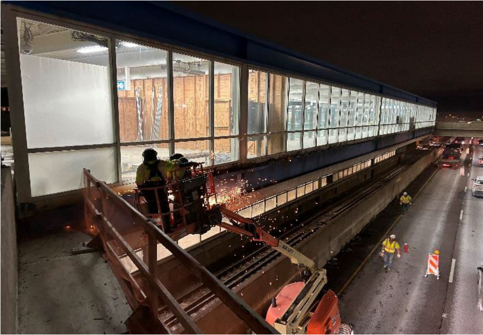
Removing Window Wash Rail from Station
