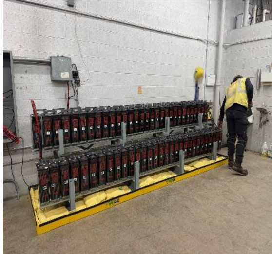
Backup Battery Installation at Damen
