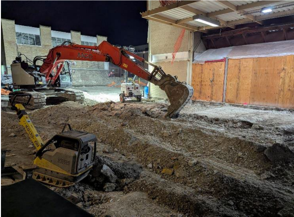
East Exit – Demolition of Pavement
