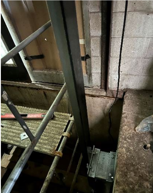
South Elevator – Framing w/ Counterweight
