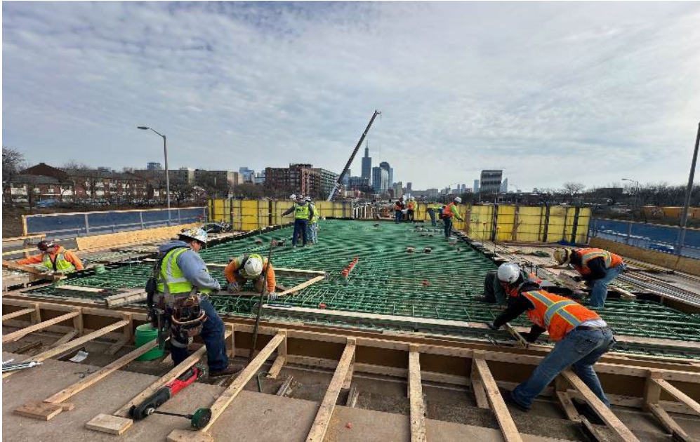
Loomis Stationhouse Deck Rebar Installation
