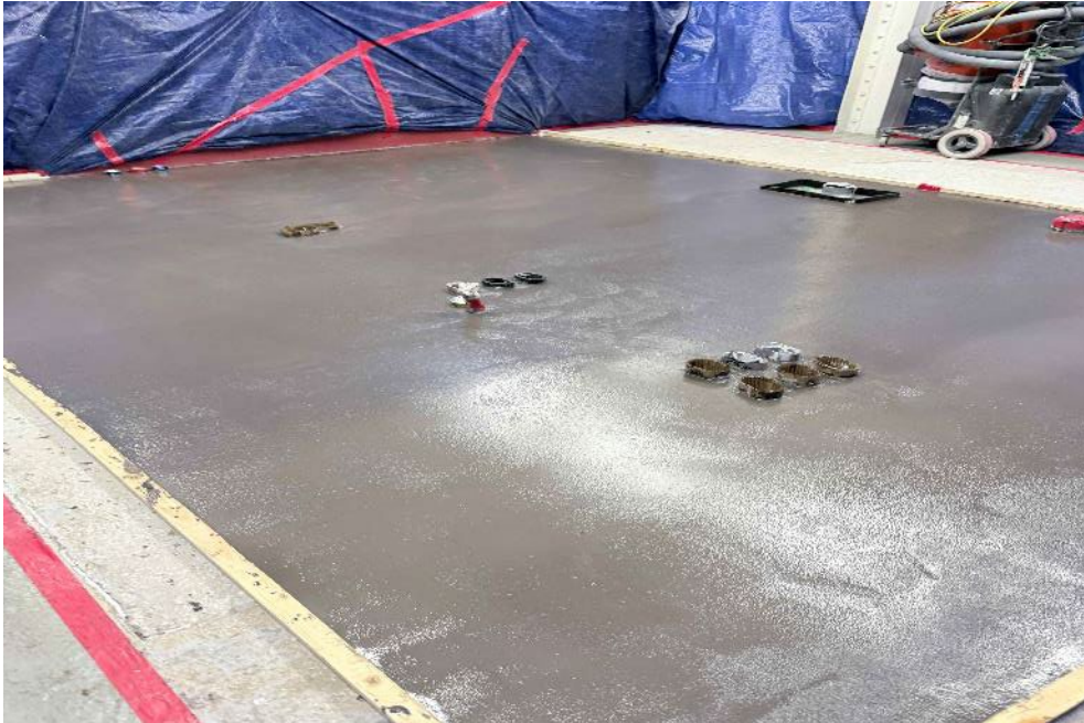
Hermitage Substation Existing Floor Leveling
