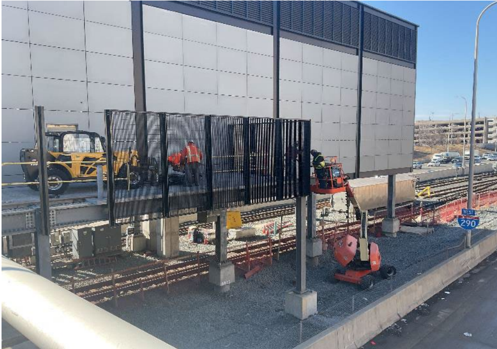
Morgan Substation Loading Dock Fence Installation
