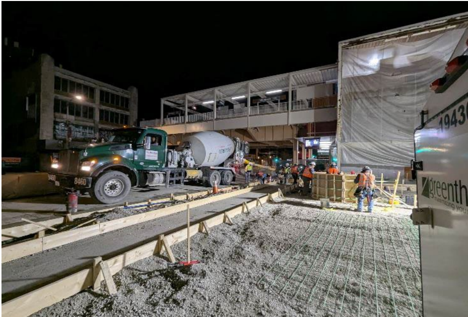
South BTA – Placing Curb and Gutter
