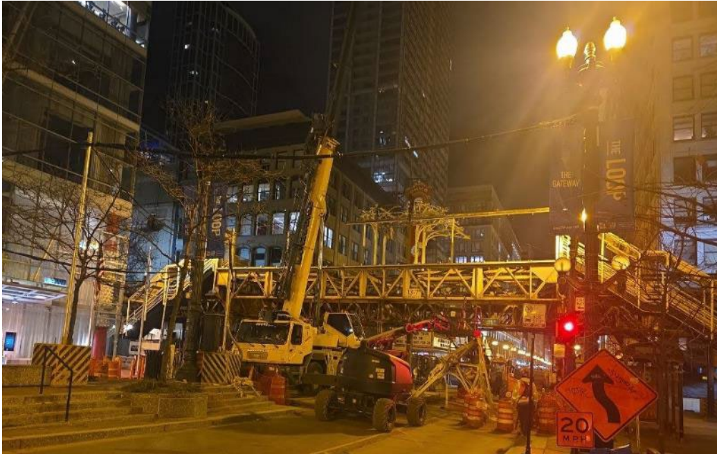
Elevated Stationhouse Demolition
