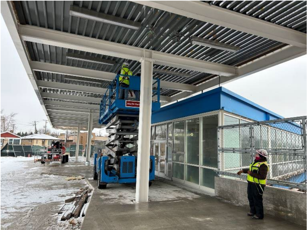
Wiring Lights at Bus Canopy
