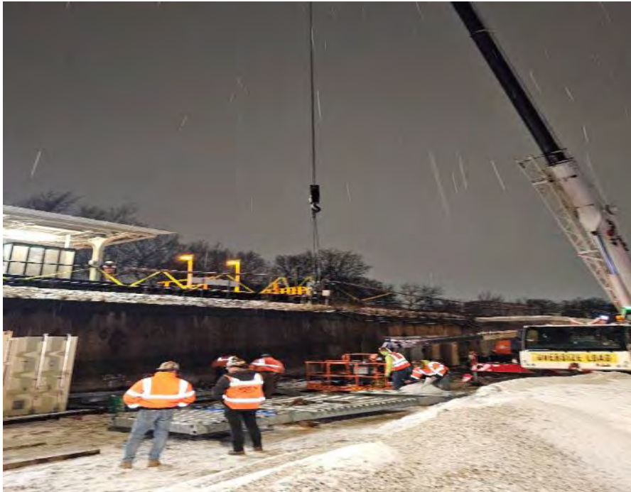
Preparing to Hoist Station House Steel Roof Framing
