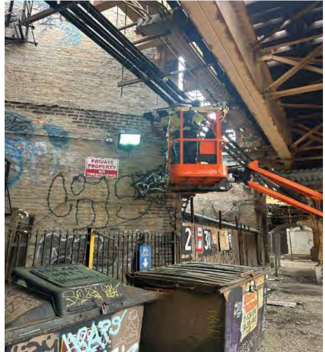
External Conduit Installation at Damen
