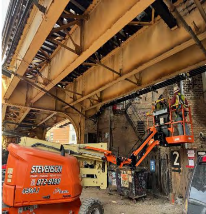
External Conduit Installation at Damen
