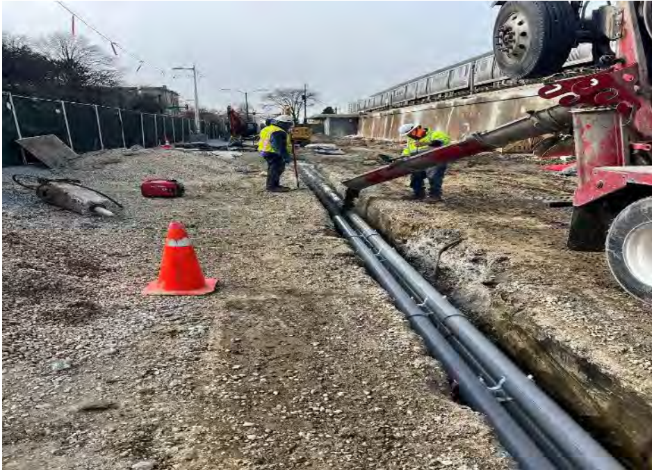
Placing Concrete Over Newly Installed Utilities
