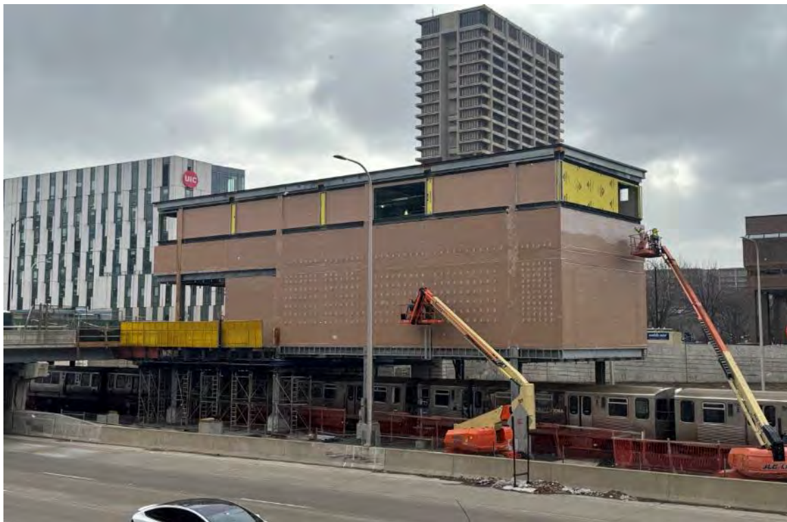
Morgan Substation HPCP Brackets & Weather Sealant
