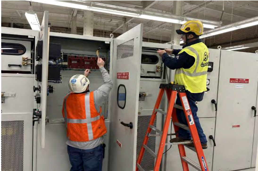
Hermitage Substation Power Lineup# 2 Removal
