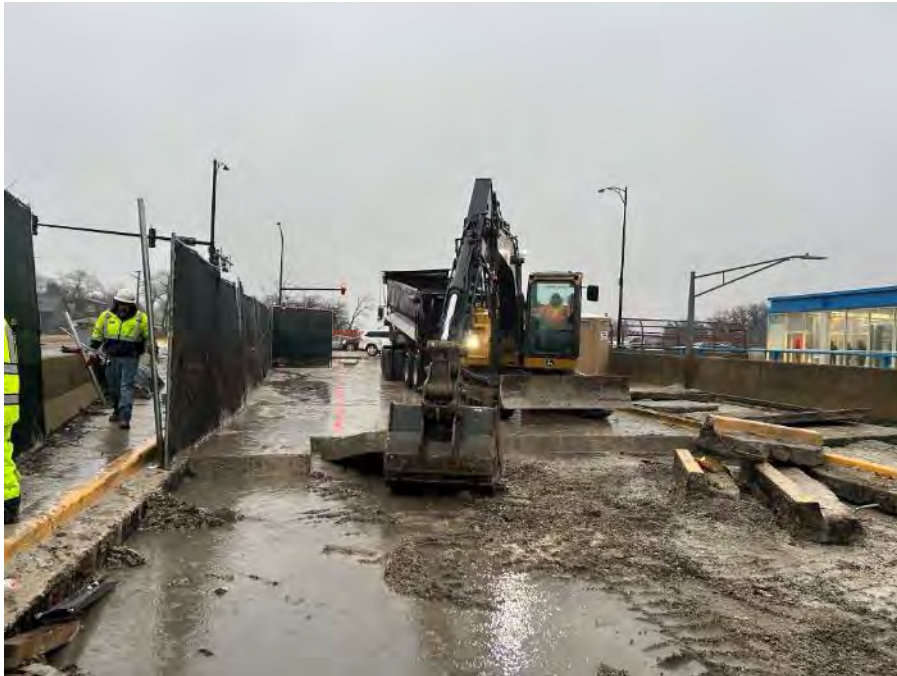
Pavement Removal at North Bridge Approach
