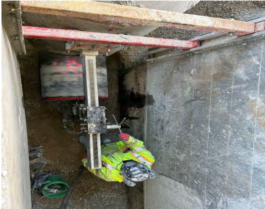
Coring 24" Hole in Manhole for sewer pipe
