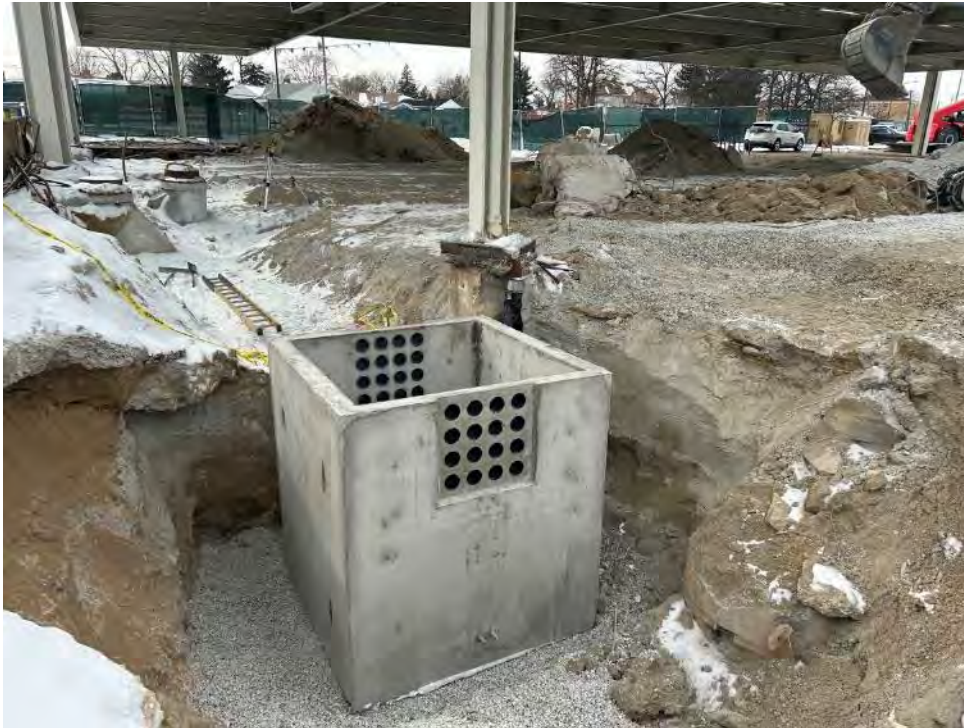
New Electrical Manhole at Bus Canopy
