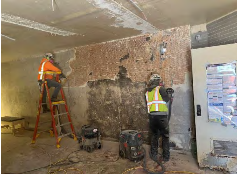
Tile Demolition at Mason Station House
