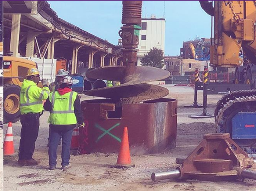
Drill new track foundations
