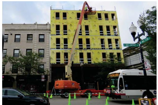
Figure 1.13: 945 W. Belmont Avenue, under construction August 2018
