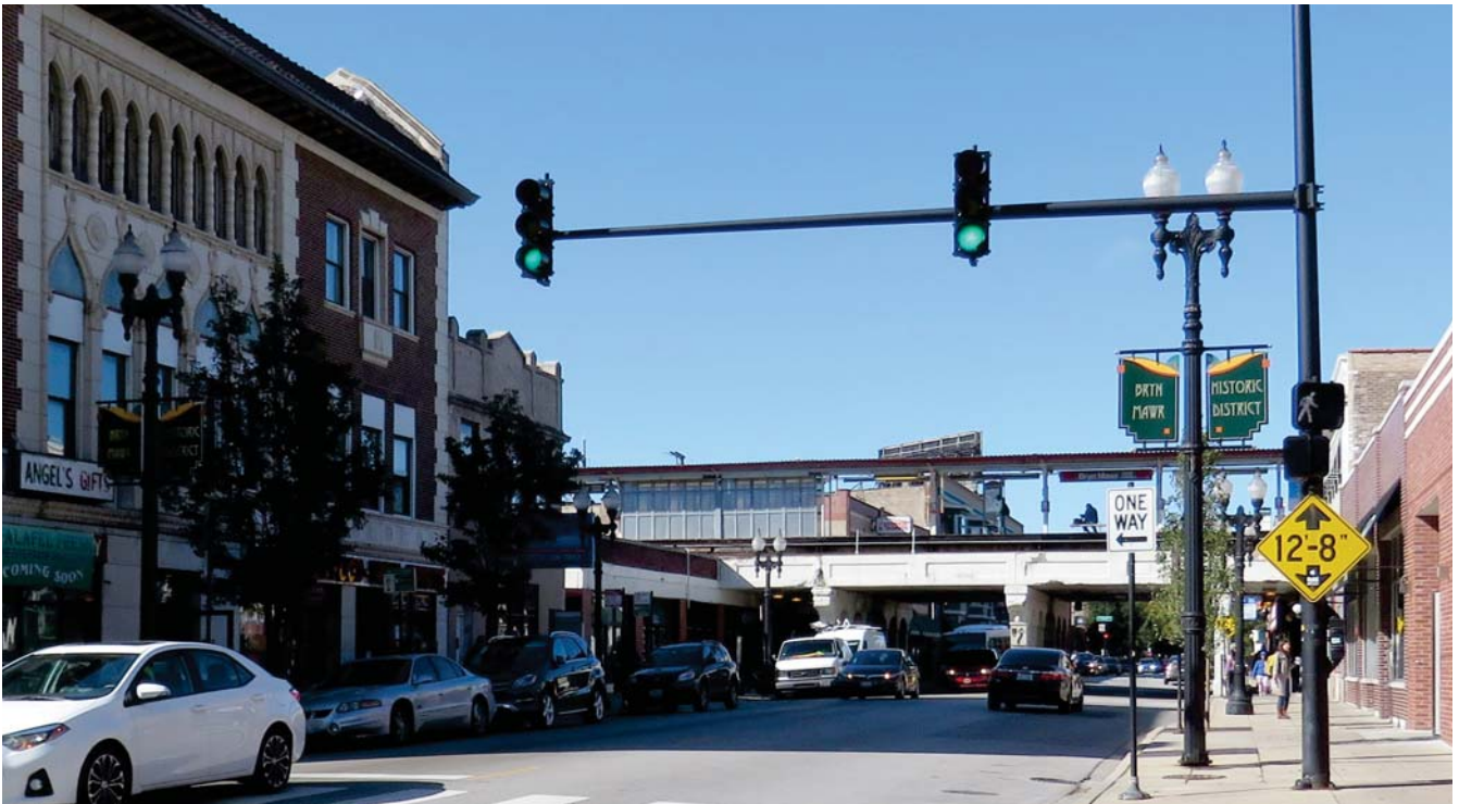
Figure 1.55: Existing condition looking west on Bryn Mawr Avenue at Winthrop Avenue
