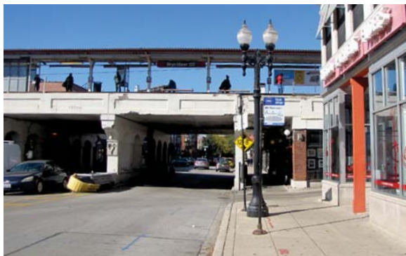
Figure 1.35: Existing columns at Bryn Mawr station
