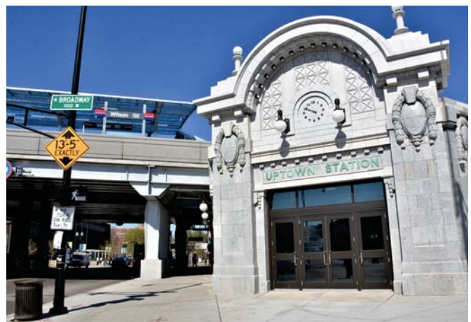
Figure 1.22: Wilson Red Line station reconstruction (2018)
