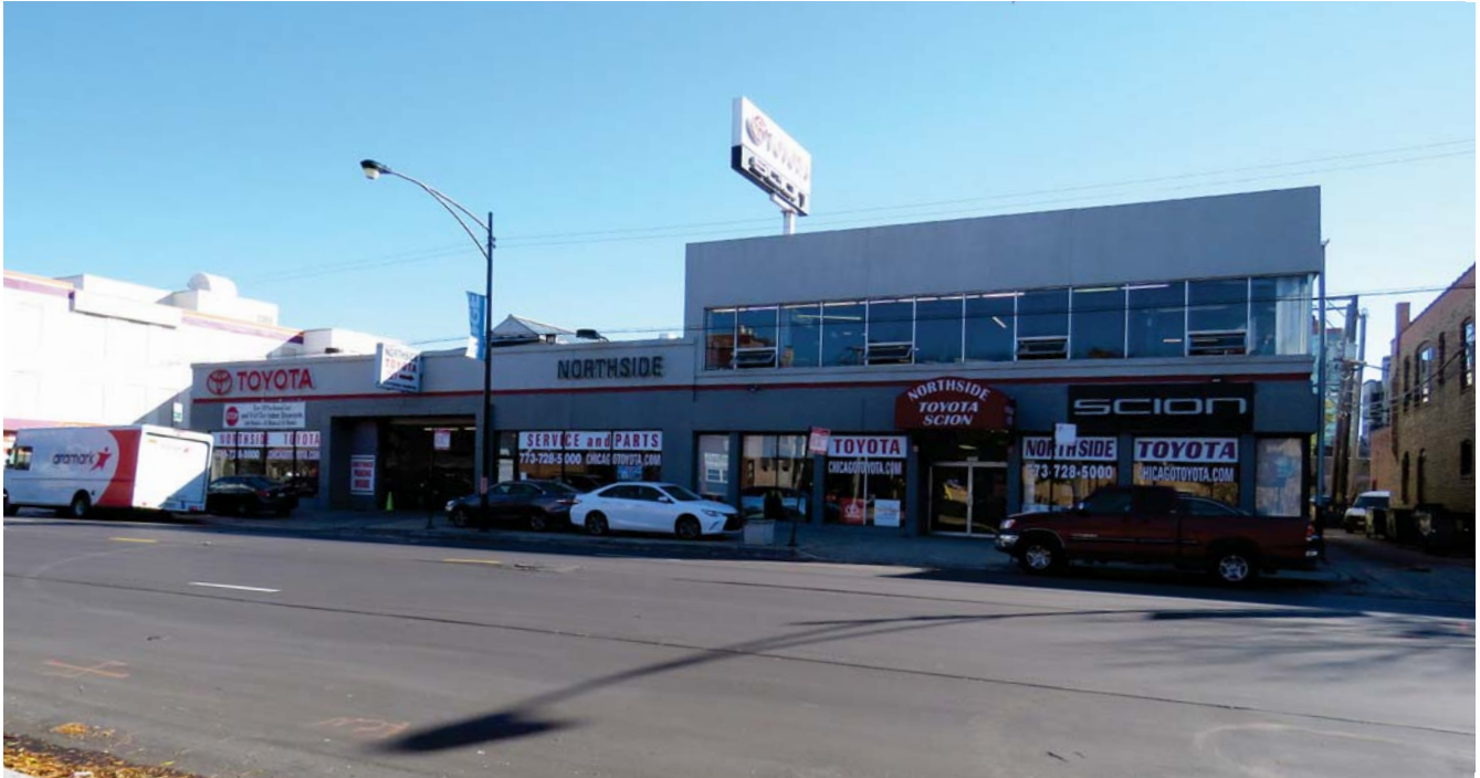
Figure 1.64: 5619-5625 N. Broadway Site, November 2016
