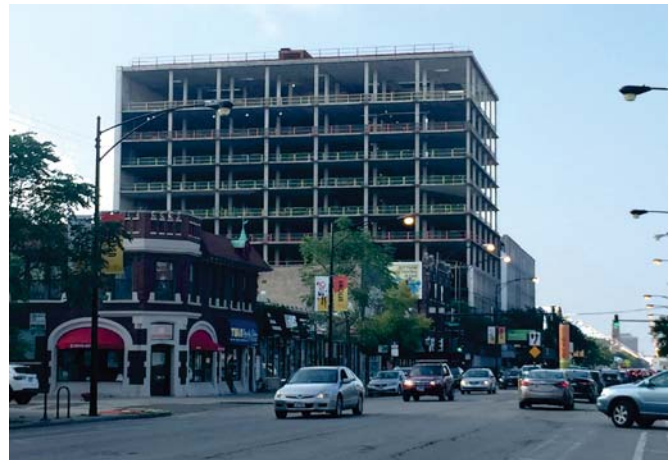
Figure 1.21: 5050 North Broadway, currently under construction
