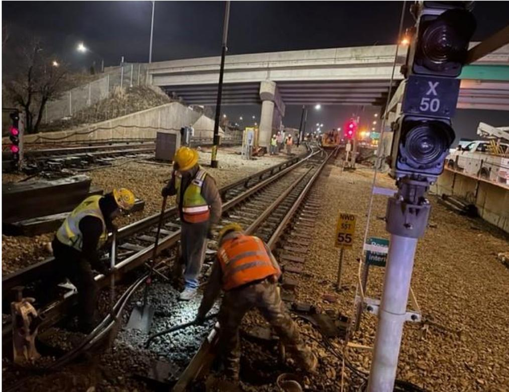
Installing ballast at trip ties
