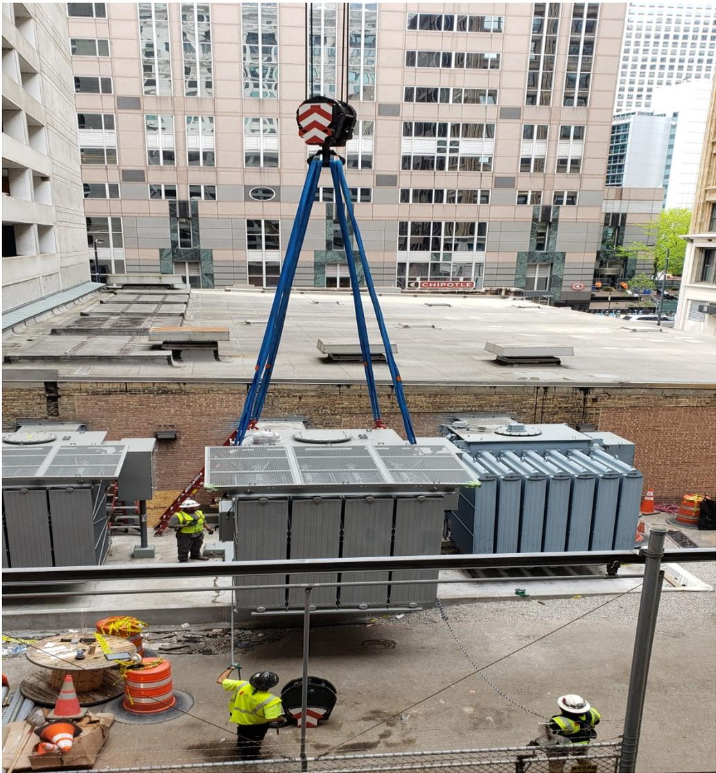
**Placing New Transformer 2 at Franklin Substation**
