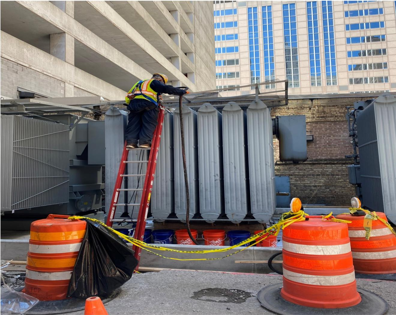
**Draining Oil and Flushing Transformer 2 at Franklin Substation**
