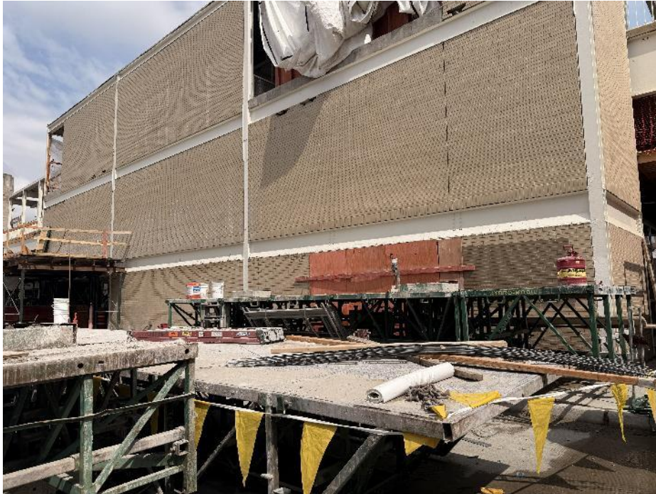
South Elevation – Completed Masonry Wall
