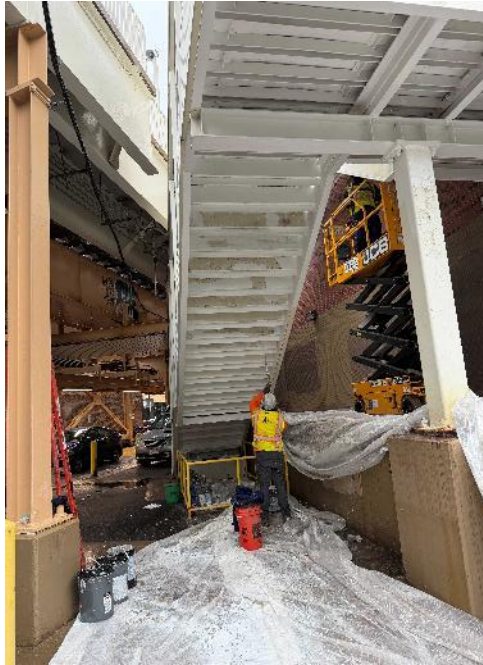
Inbound Exit Stair – Prep and Paint
