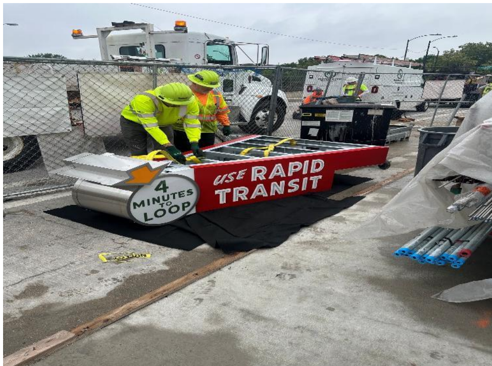
Loomis Stationhouse Storefront Historical Sign
