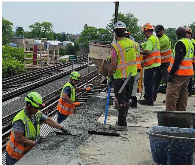
Halsted/63 rd - Tactile Repair
