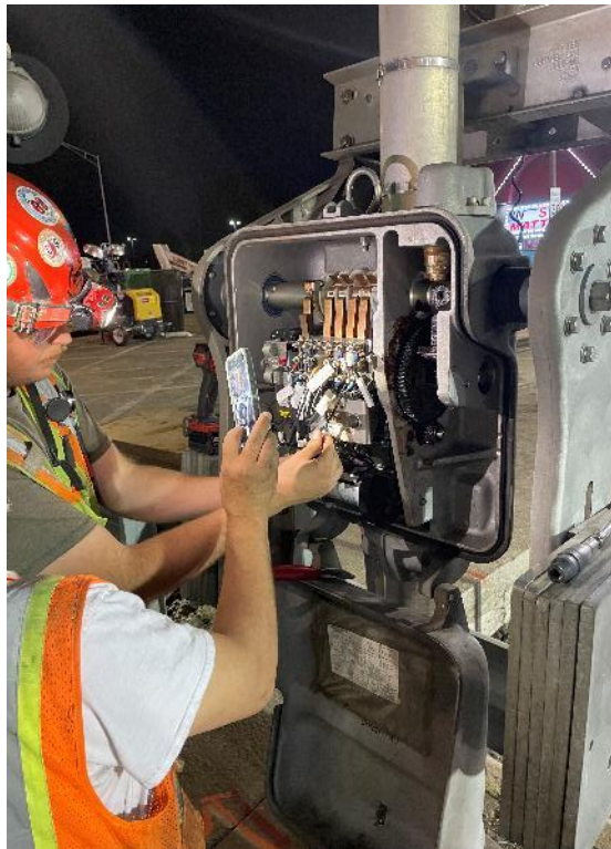
Crossing Gate Mechanism Replacement
