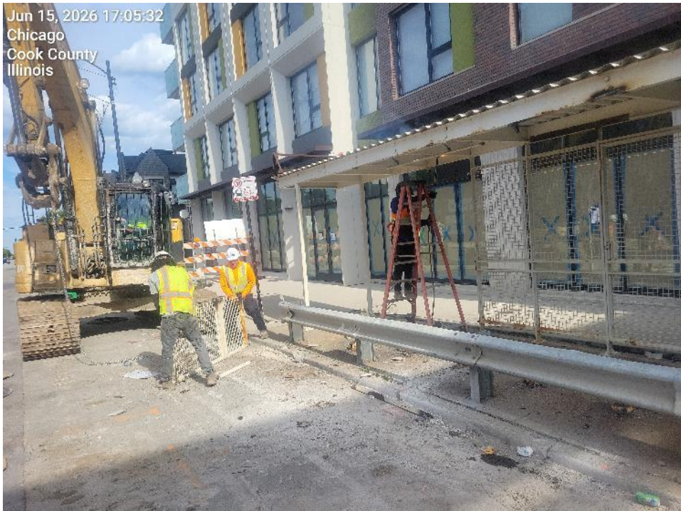
SE Exit Stair – Demolition of Old Canopy
