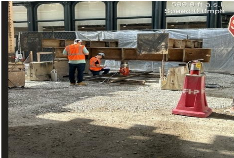
State Street Bent Compression Testing
