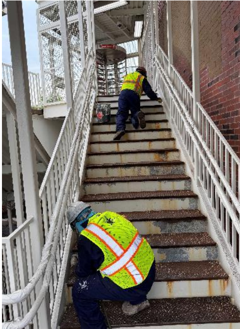
Inbound Exit Stair – Prep and Paint
