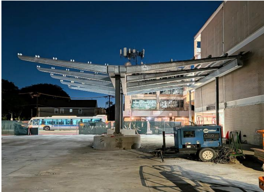
South BTA – Structural Steel Progress
