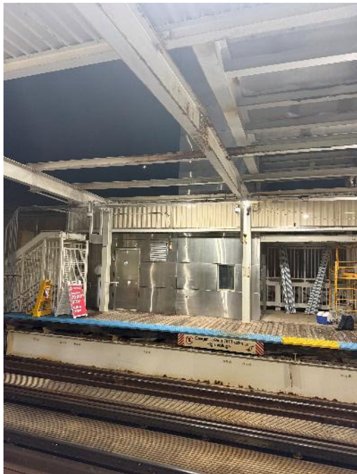
East Canopy – Demolition of Corrugated Roofing
