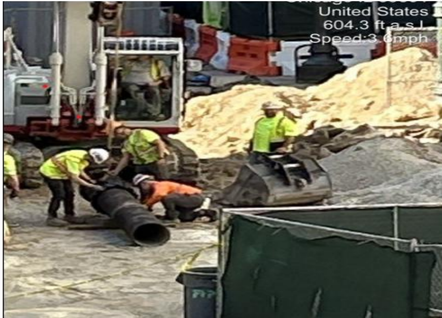
Installation of Pipe north of State Street
