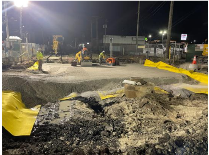
Installation of Geofabric and Sub-base
