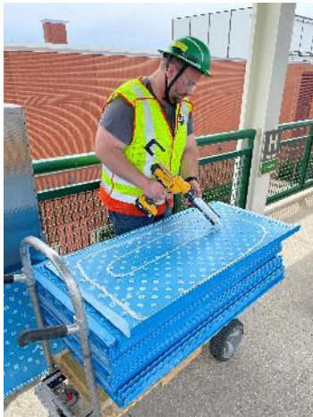
Halsted/63 rd - Tactile Repair
