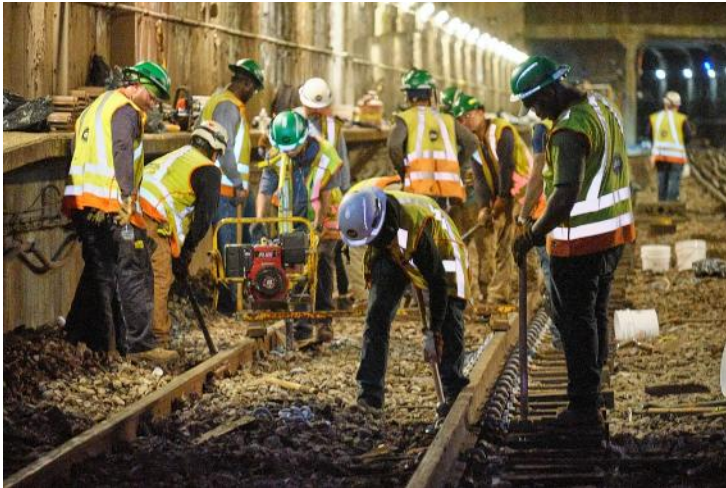
Track Workers installing plates and fasteners on new ties
