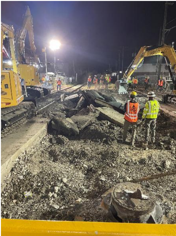
Demolition of Existing Track
