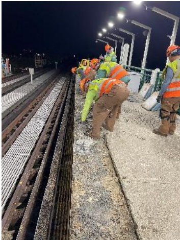
Halsted/63 rd - Tactile Repair
