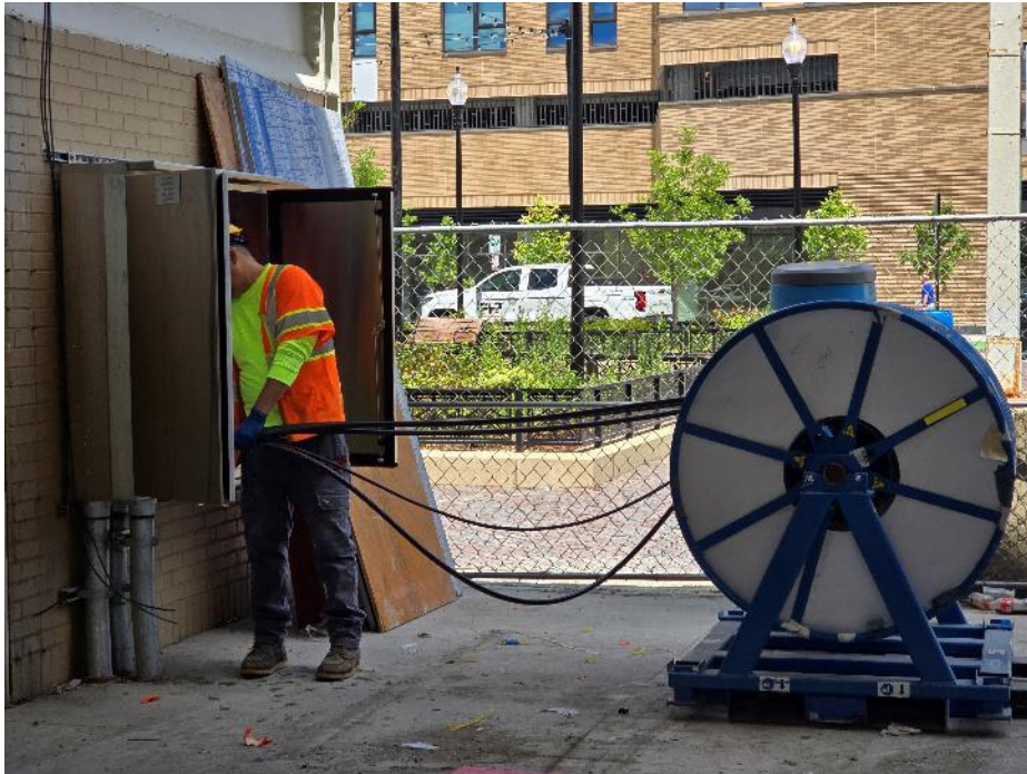
Pulling Electric Cable to Electric Room
