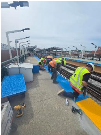
Halsted/63 rd - Tactile Repair
