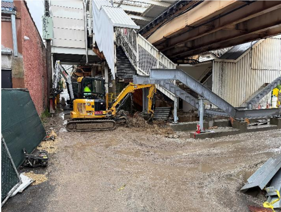
Demolition – Inbound Main Stair
