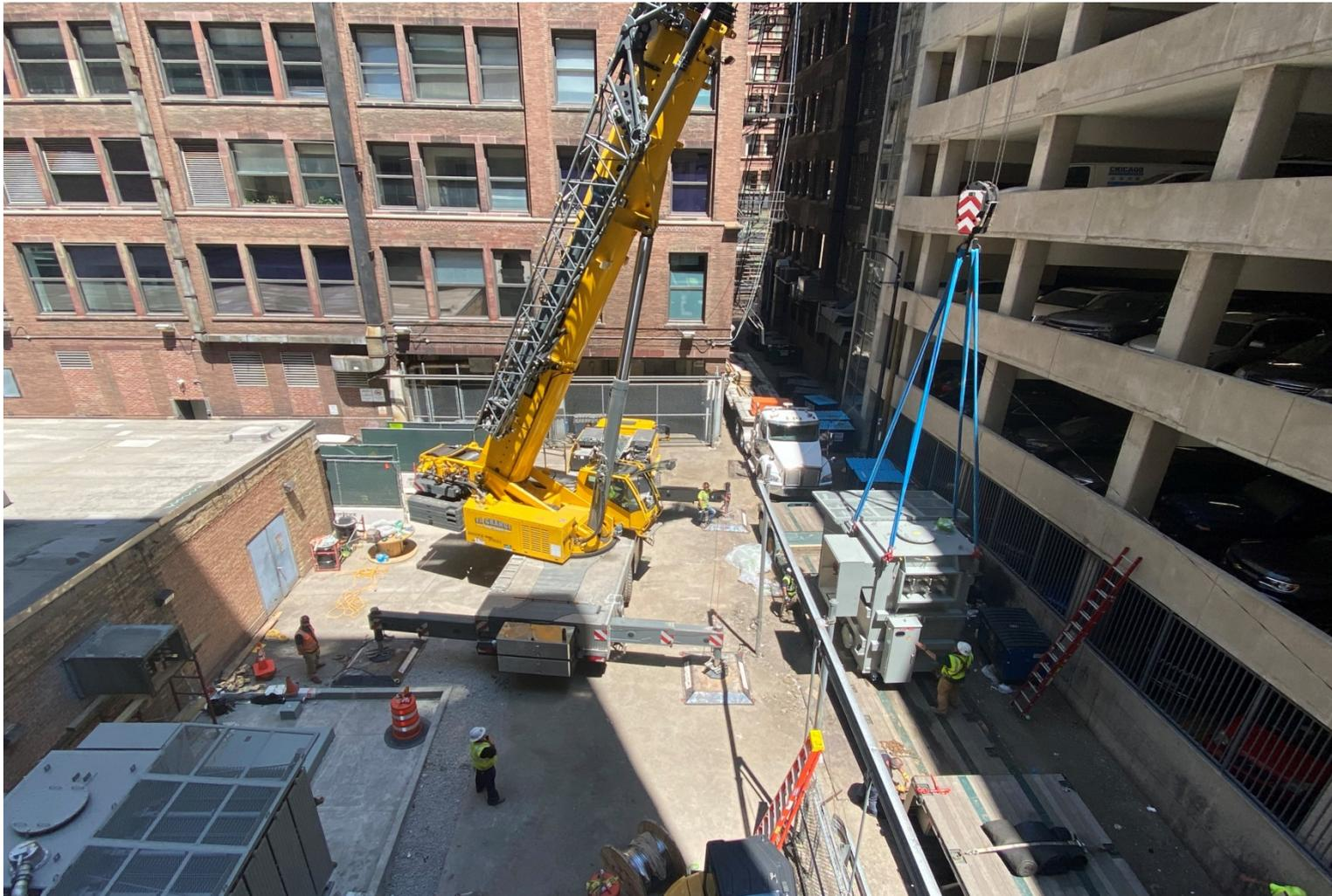
**Lifting and Placing New Transformer 3 at Franklin Substation**
