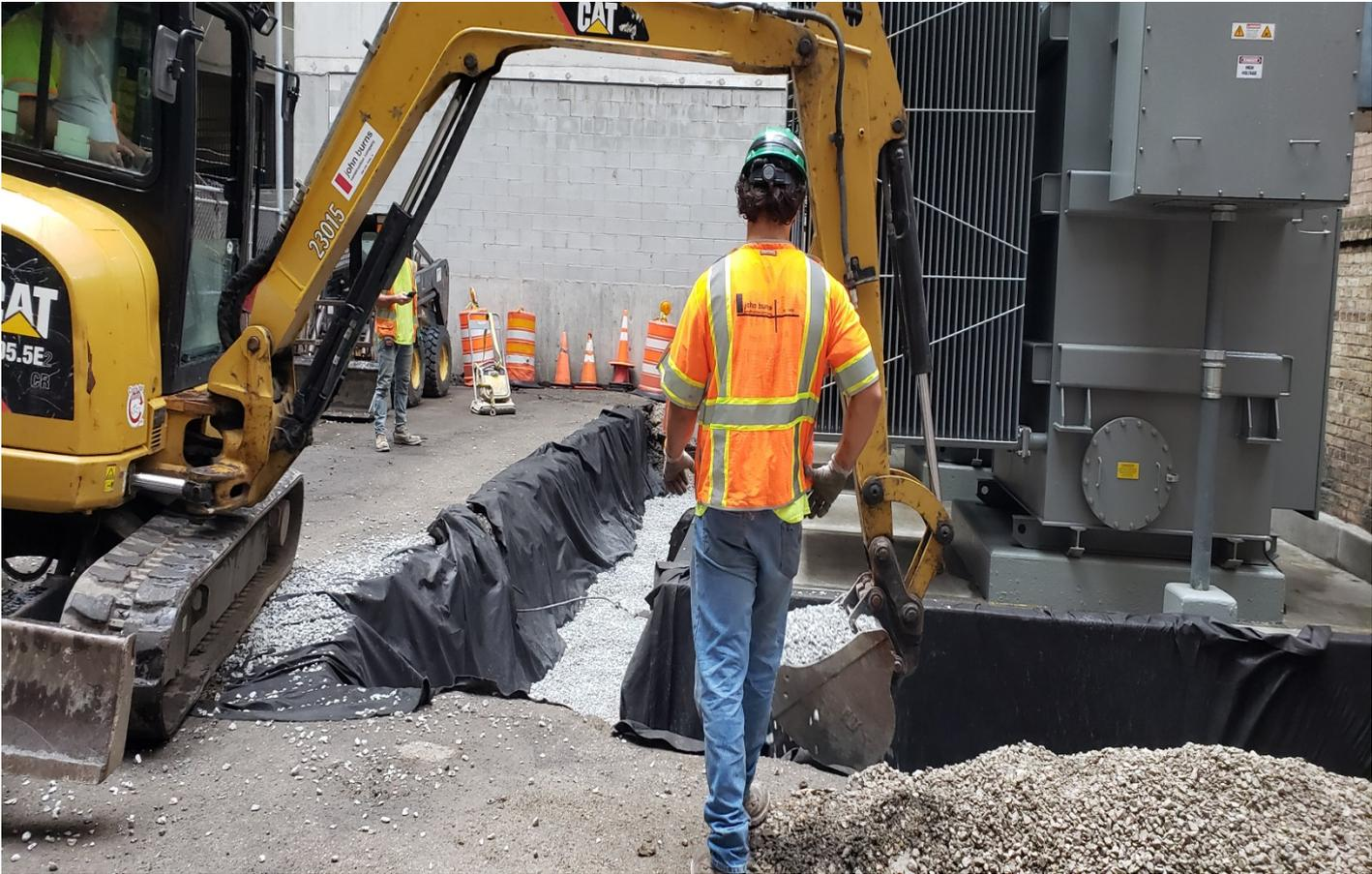
**Re-filling Stone Around The Concrete Containment Pad**
