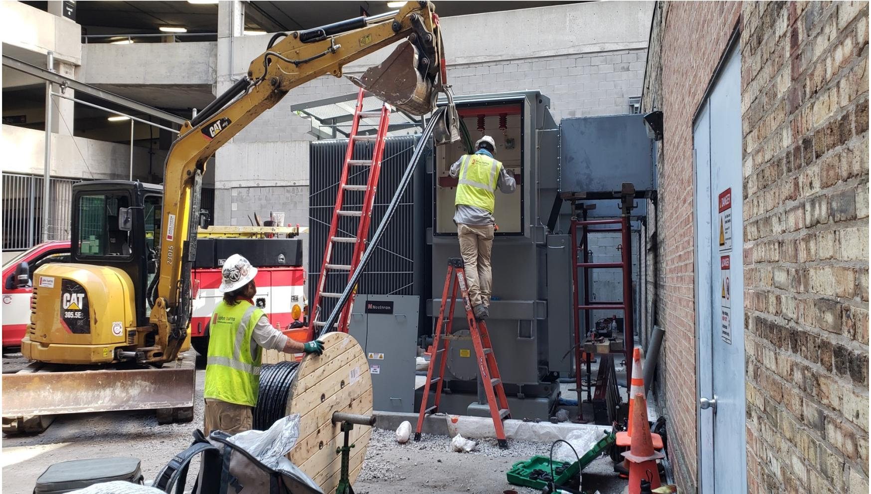
**Cable Pull Between the AC/DC Gears and the New Transformer 3
