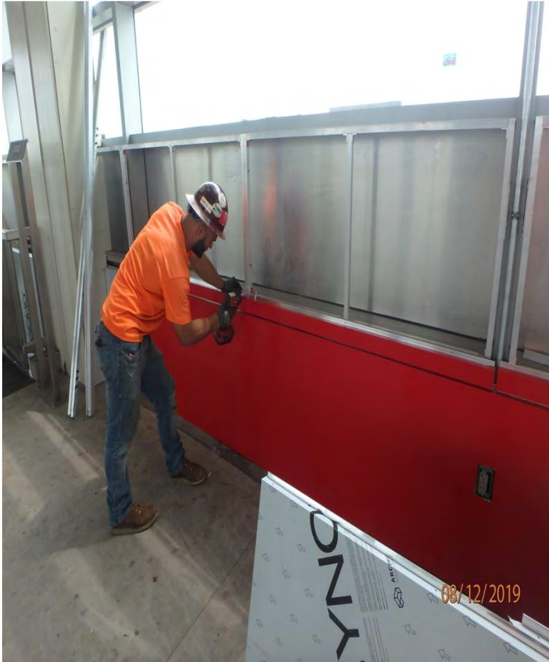
**Installing Interior red-panels at the Pedestrian Bridge**
