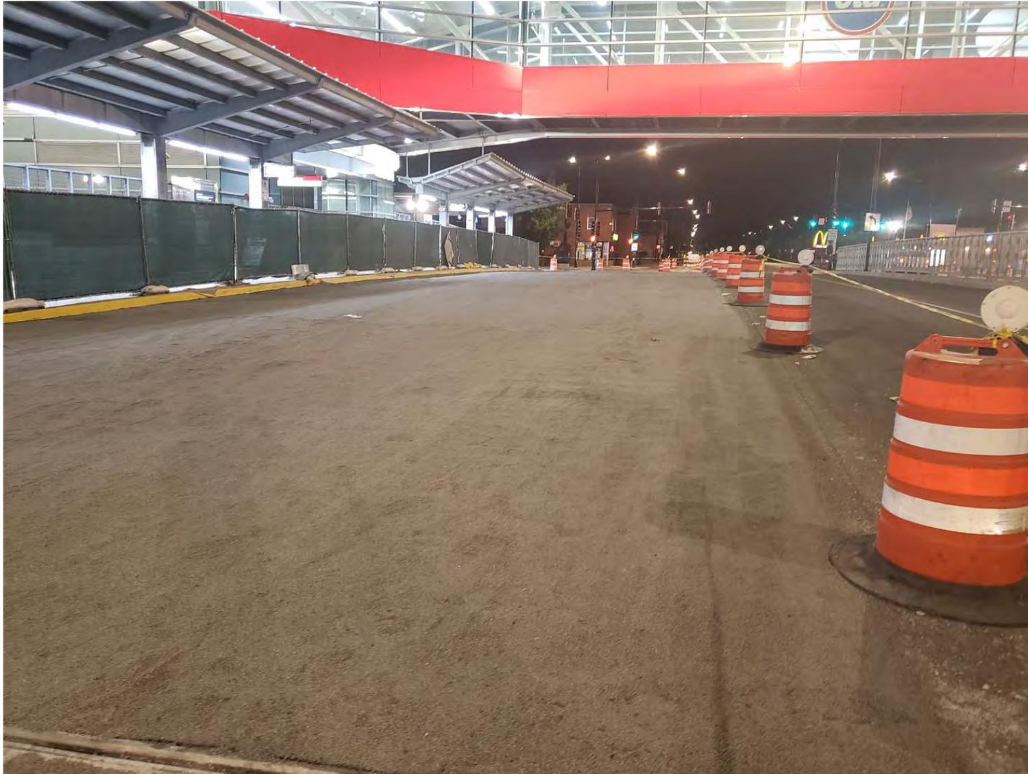
**Finished Polymer Overlay On EB of 95<sup>th</sup> Bridge**
