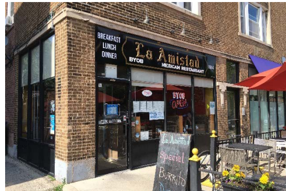
Example of an inappropriate contemporary storefront alteration not in the district. The original storefront would have been recessed.
