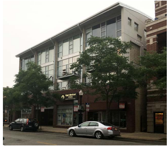
Example of an inappropriate rooftop addition located outside of the district. This rooftop addition maintained the building's pedestrian-scale by preserving the historic ground floor storefront, but is incompatible with the historic building due to its scale, and contemporary design, and materials.
