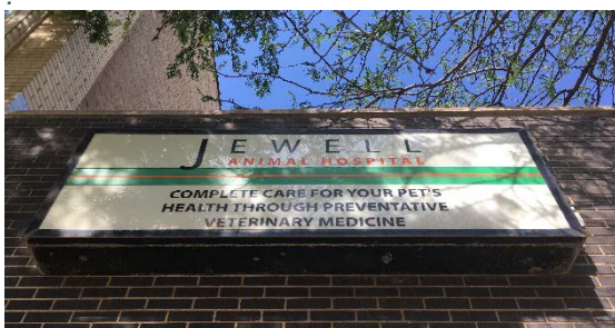
Example of an inappropriate box sign not in the district. This sign is not integrated into the design of the building, obscures a larger portion of the main façade, and is mounted directly into the brick.
