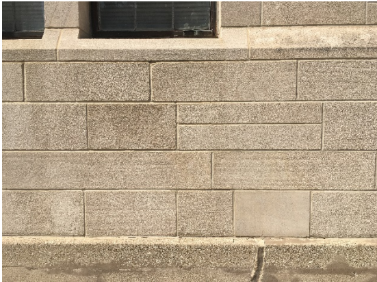
Example of typical limestone cladding in the district.
