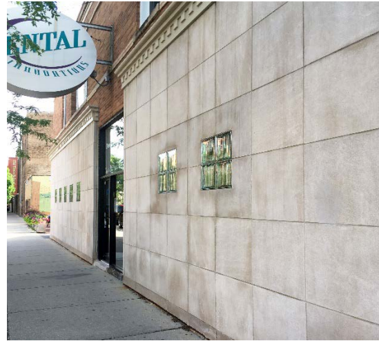
Example of an inappropriate, contemporary storefront alteration not in the district. Incompatible limestone veneer has been applied to the original storefront and glass block windows installed which are disproportionate in size, type, and material.
