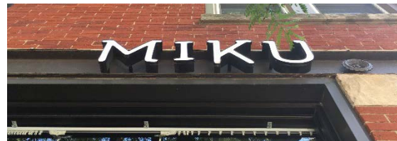
Example of inappropriate sign mounting, located outside of the district, as the sign is directly attached to the historic cast iron header.
