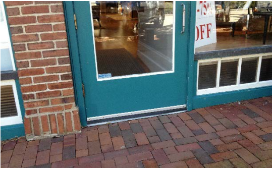
Example of an ADA-compliant threshold not in the district.
