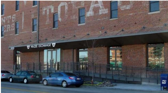
Example of an appropriate contemporary exterior ramp at a side entrance not in the district.
