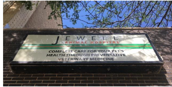
Example of an inappropriate box sign not in the district. This sign is not integrated into the design of the building, obscures a larger portion of the main façade, and is mounted directly into the brick.
