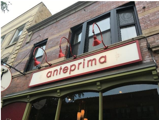
Example of inappropriate gooseneck exterior lighting and exposed conduit not in the district.
