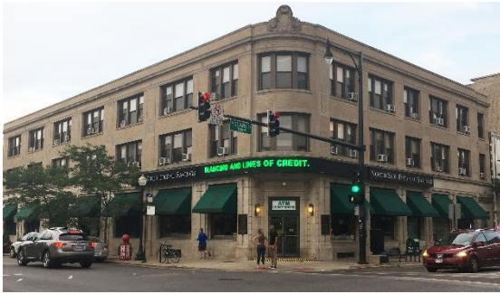
Example of an inappropriate digital banner sign not in the district, that is directly mounted into the building's limestone cladding and obscures architectural features at the first floor.
