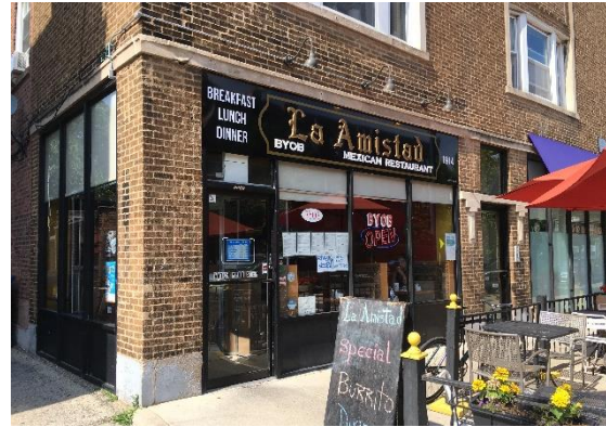
Example of an inappropriate contemporary storefront alteration not in the district. The original storefront would have been recessed.
