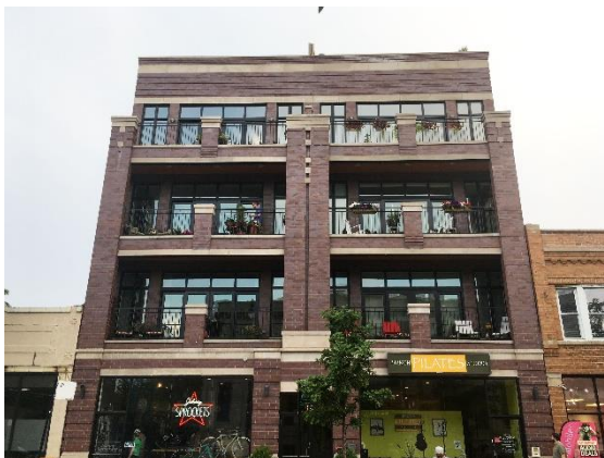
Located outside of the district, this new infill construction maintained the pedestrian-scale of the neighborhood through the incorporation of storefronts at the first floor. It uses compatible materials, but is disproportionate in scale and massing to its surroundings.
