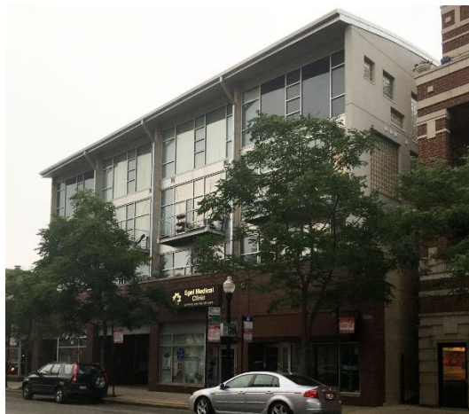
Example of a rooftop addition, located outside of the district, that maintained the building's pedestrian-scale by preserving the historic ground floor storefront, but is incompatible with the historic building due to its scale, and contemporary design and materials.
