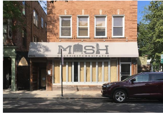
Example of an incompatible alteration to the storefront design and window type not in the district.
