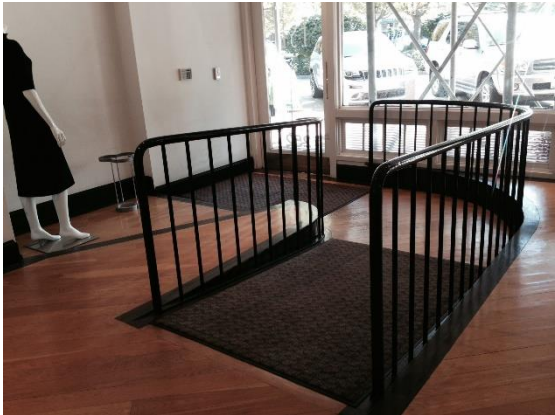
Example of an appropriate contemporary interior ramp within a retail space not in the district.
