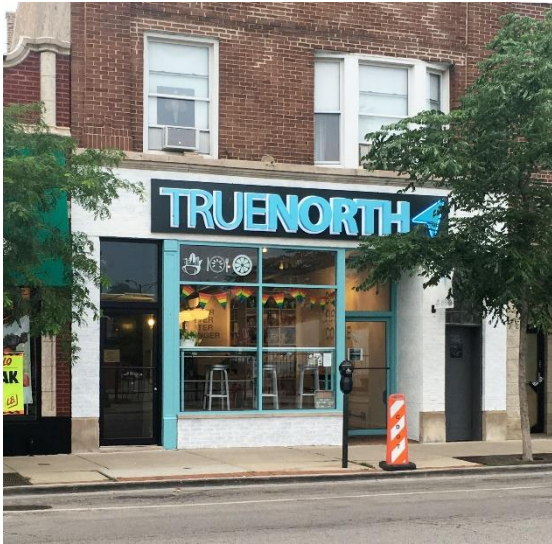
Example of a storefront, located outside of the district. It is inappropriate due to the painted brick cladding and reconfigured storefront, but has preserved some original elements, including the brick and limestone bulkhead and a cast iron column (painted blue).
