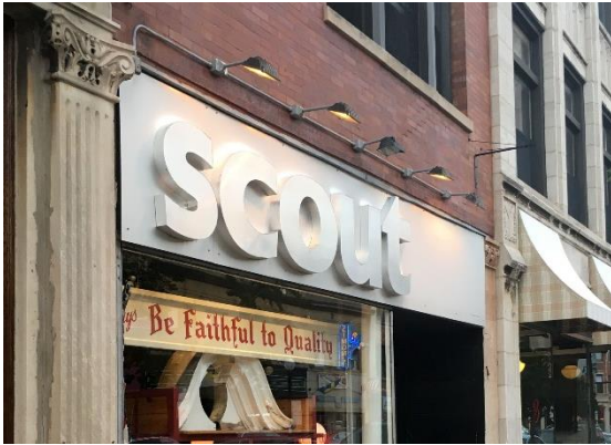
Example of an inappropriate contemporary sign not in the district. The letters are disproportionately scaled and obscure the historic storefront/transom configuration.
