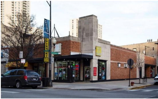
Example of an intact mid-twentieth century storefront with few contemporary alterations in the district
