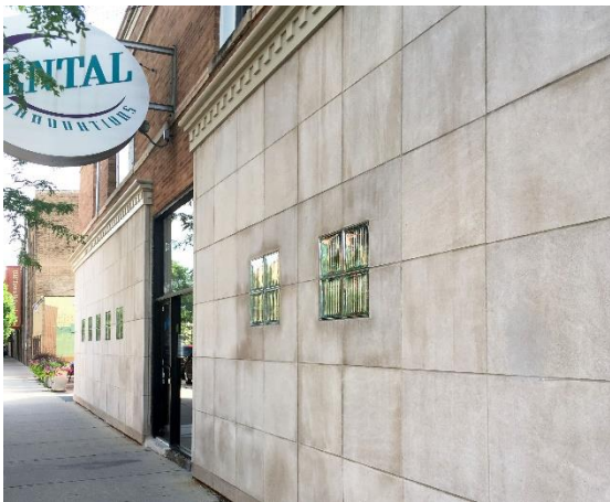
Example of an inappropriate, contemporary storefront alteration not in the district. Incompatible limestone veneer has been applied to the original storefront and glass block windows installed which are disproportionate in size, type, and material.
