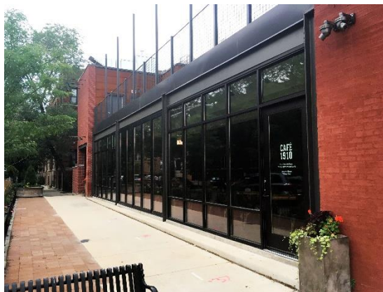
Example of appropriate contemporary rear addition not in the district. It uses contemporary materials and respects the overall scale and shape of the historic building.
