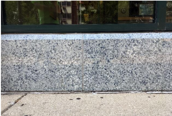
Example of granite cladding in the district.
