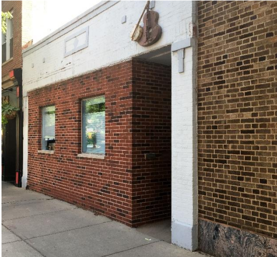
Example of an inappropriate contemporary storefront alteration, outside of the district, where the historic storefront has been infilled with brick.
