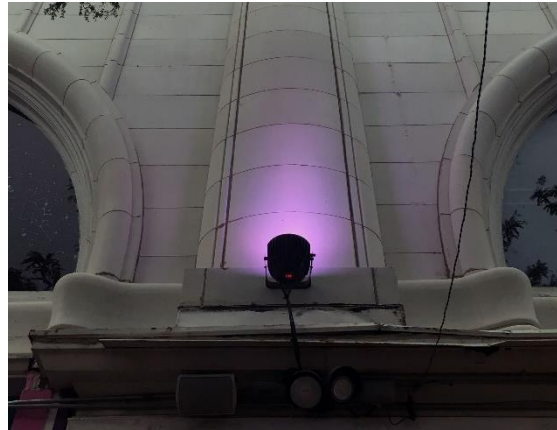
Example of contemporary architectural lighting, located outside of the district, that appropriately lights an architectural feature, but is not concealed.
