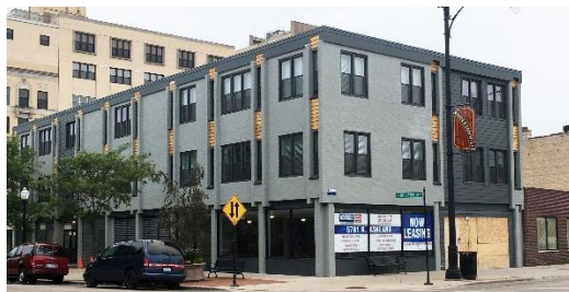
Located outside of the district, this new infill construction maintains an appropriate scale and massing and rhythm of the storefront at the first floor, but uses inappropriate materials such as painted brick and wood shakes and siding.
