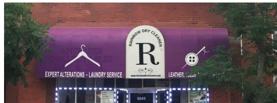
Example of an inappropriate contemporary "waterfall" awning, located outside of the district.
