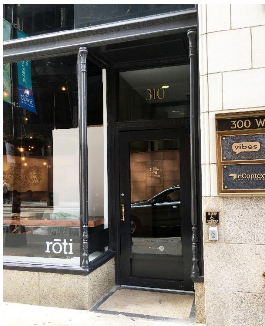
Example of a contemporary door type that is appropriate to this historic building not in the district.
