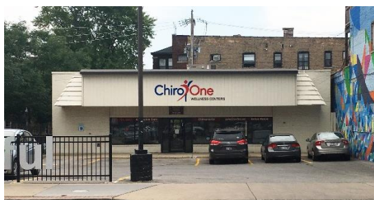
Example of inappropriate non-historic construction not in the district. The building is disproportionate in scale and massing to its surroundings and setback from the street.
