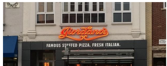
Example of appropriate contemporary signage, located outside of the district, that is appropriately attached into the mortar joints and not the masonry façade of the building.
