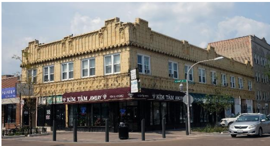
Example of a typical Two-Part Commercial Block in the district.
