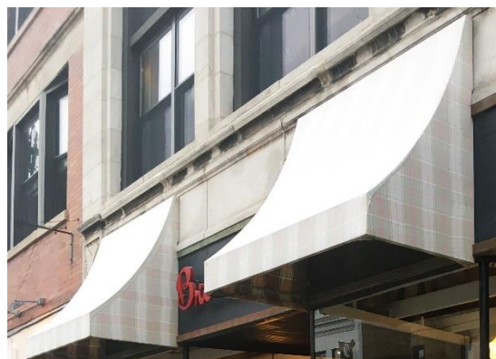
Example of an inappropriate contemporary "concave" awning, located outside of the district.
