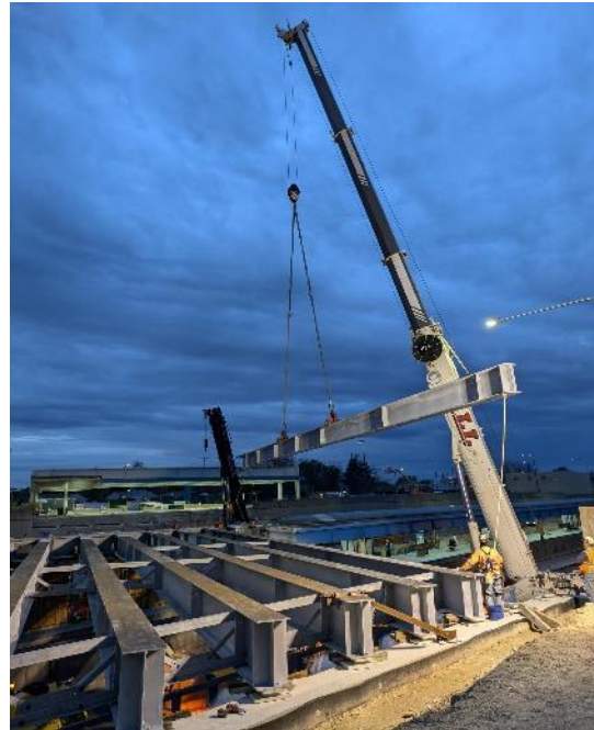
Lifting Steel Beams over NB
