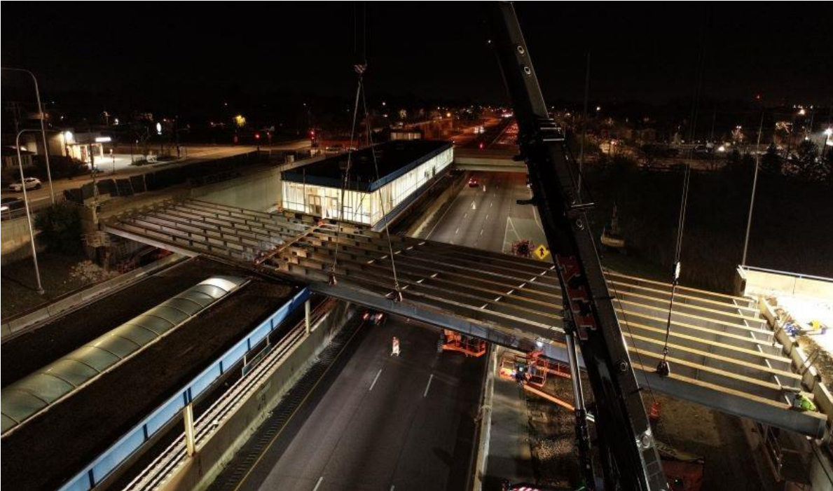
Lifting Last Beam over Inbound I-90 at Night
