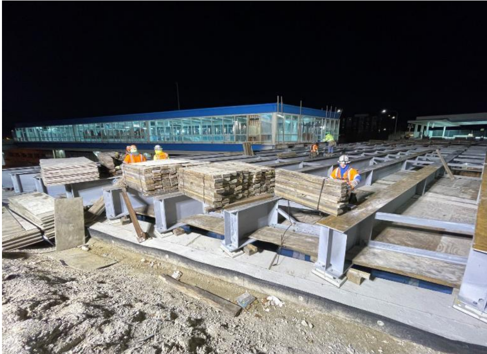
Installing Protective Shielding Between New Beams
