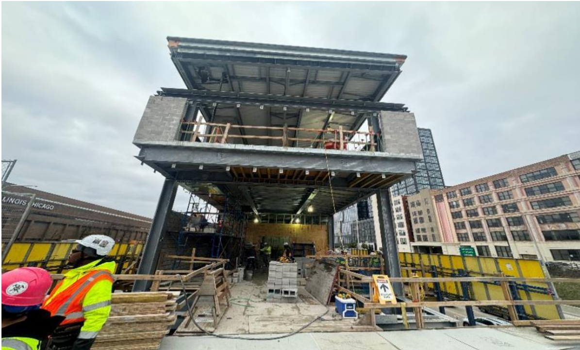
Morgan Substation Bridge Level View
