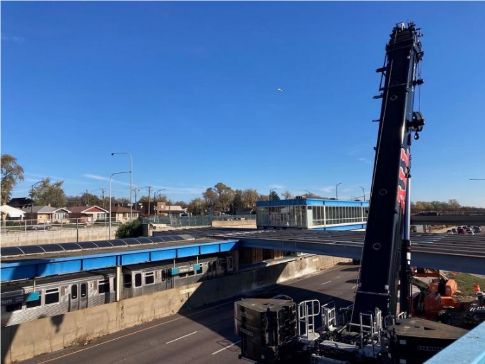
Completed Steel Beam Installation
