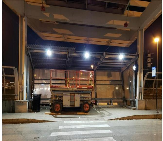
**47<sup>th</sup> Red Line – Install directional flood lightening on steel structure to illuminate bus stop waiting area**
