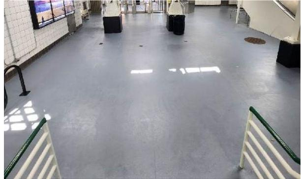
**51<sup>st</sup>/Green Line – Paint station floor with grey epoxy paint**
