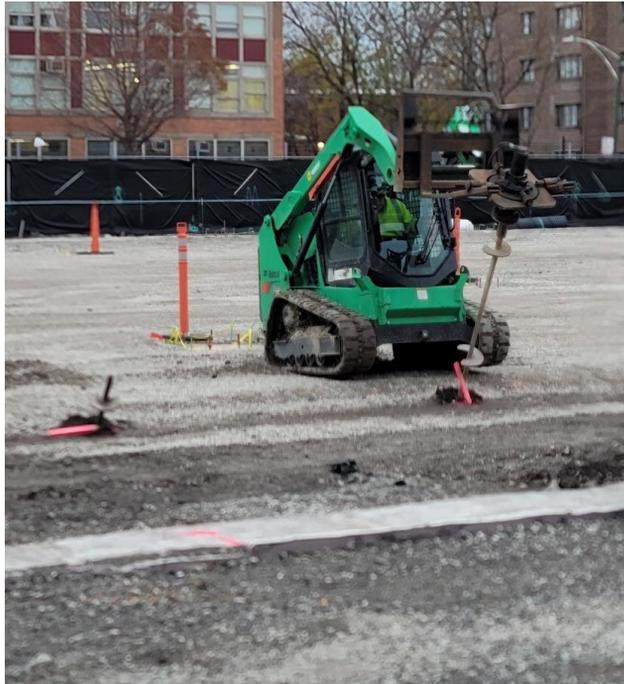
**Helical Anchor Installation for Precast Support**
