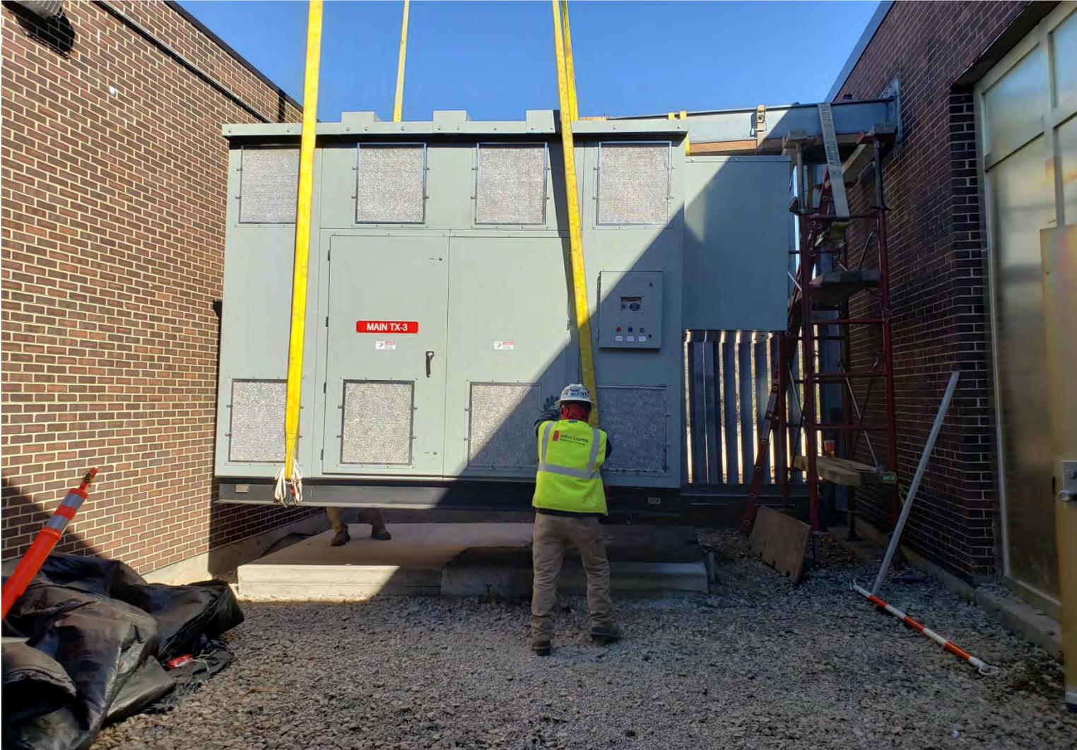
**Setting New Transformer# 3 at Edmunds Substation**
