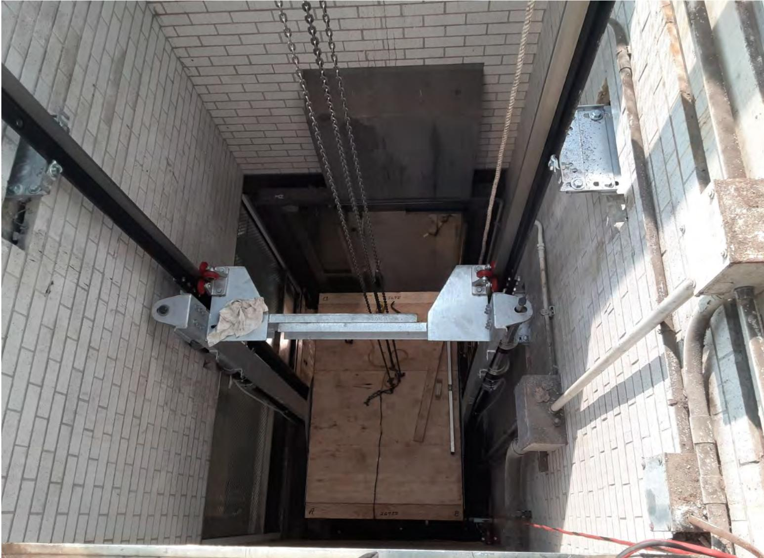
**Elevator #2 – New Elevator Rails and Cab Floor Installation**
