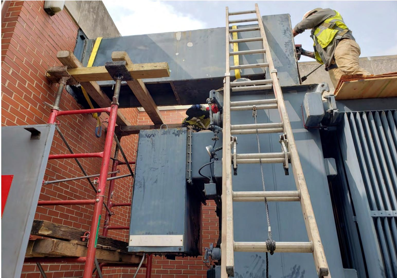
**Assembling Scaffolding to Support Existing Anode Bus for Transformer 3 at Lotus Substation**
