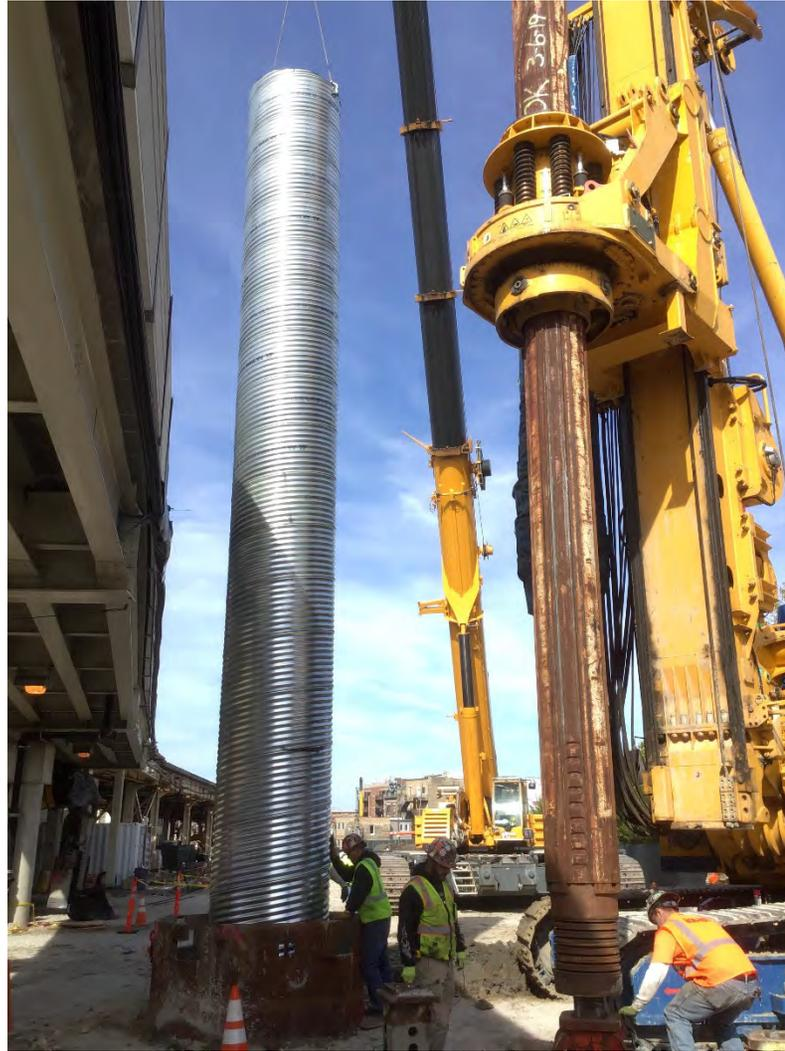
**Red-Purple Bypass – Installing Permanent Liner in Drilled Shaft**
