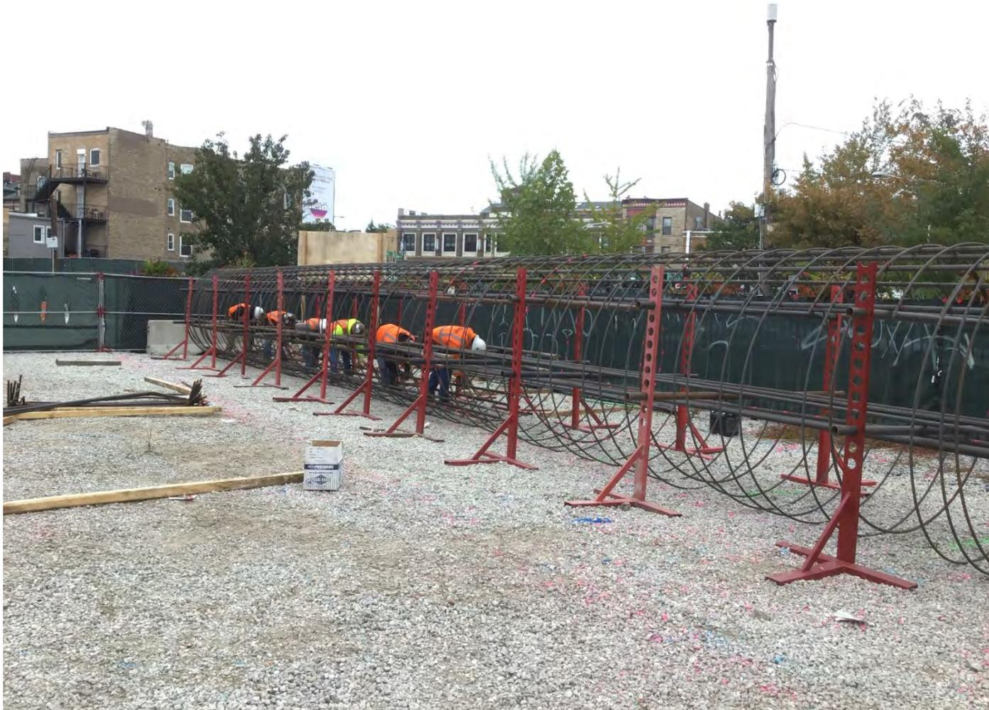
**Red-Purple Bypass – Assembling Rebar Cage for Drilled Shaft**
