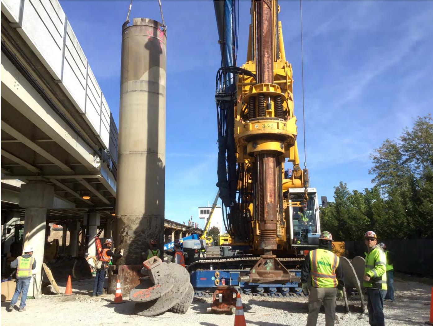
**Red-Purple Bypass – Placing Temp Steel Casing in Drilled Shaft**
