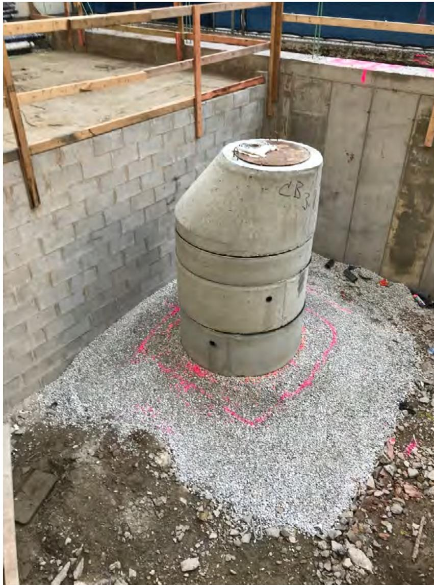
**Catch Basin Installation in Courtyard at East Lake Substation**
