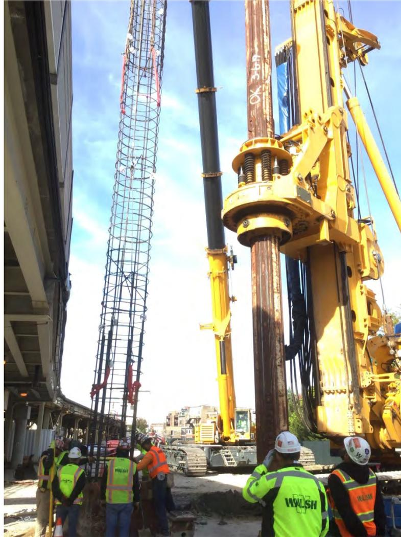
**Red-Purple Bypass – Installing Rebar Cage in Drilled Shaft**
