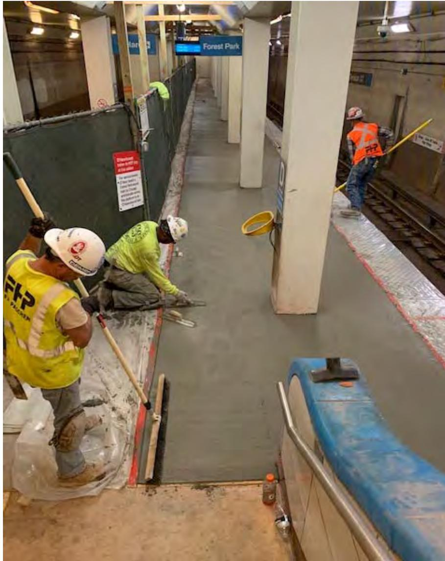
**Finishing of Division Station SB Platform Concrete Topping**
