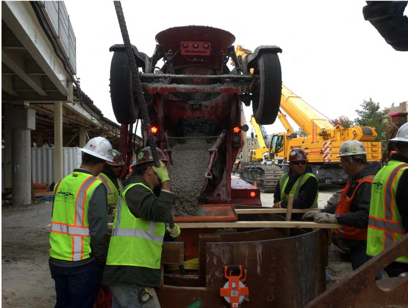
**Red-Purple Bypass – Placing Concrete via Tremie Pipe in Drilled Shaft**
