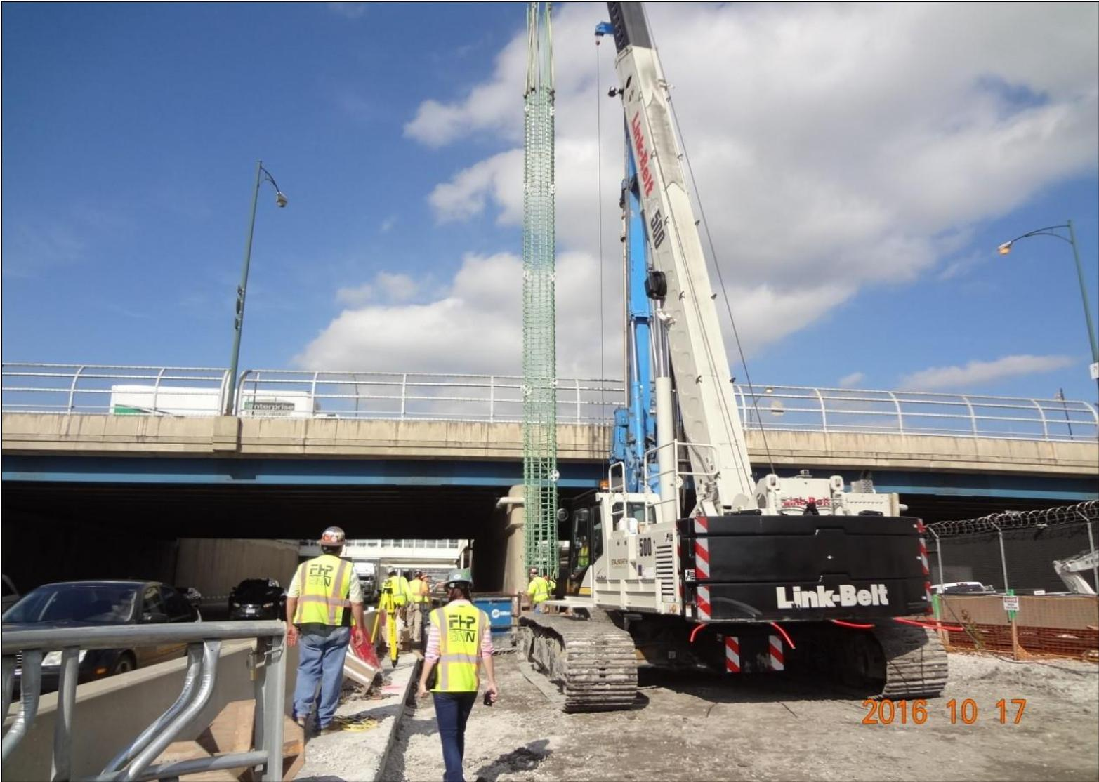
**Rebar Installation for South Terminal Caissons**
