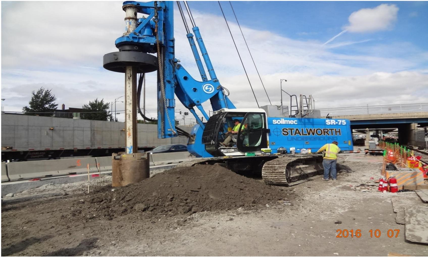
**South Terminal Caisson Foundation Drilling**
