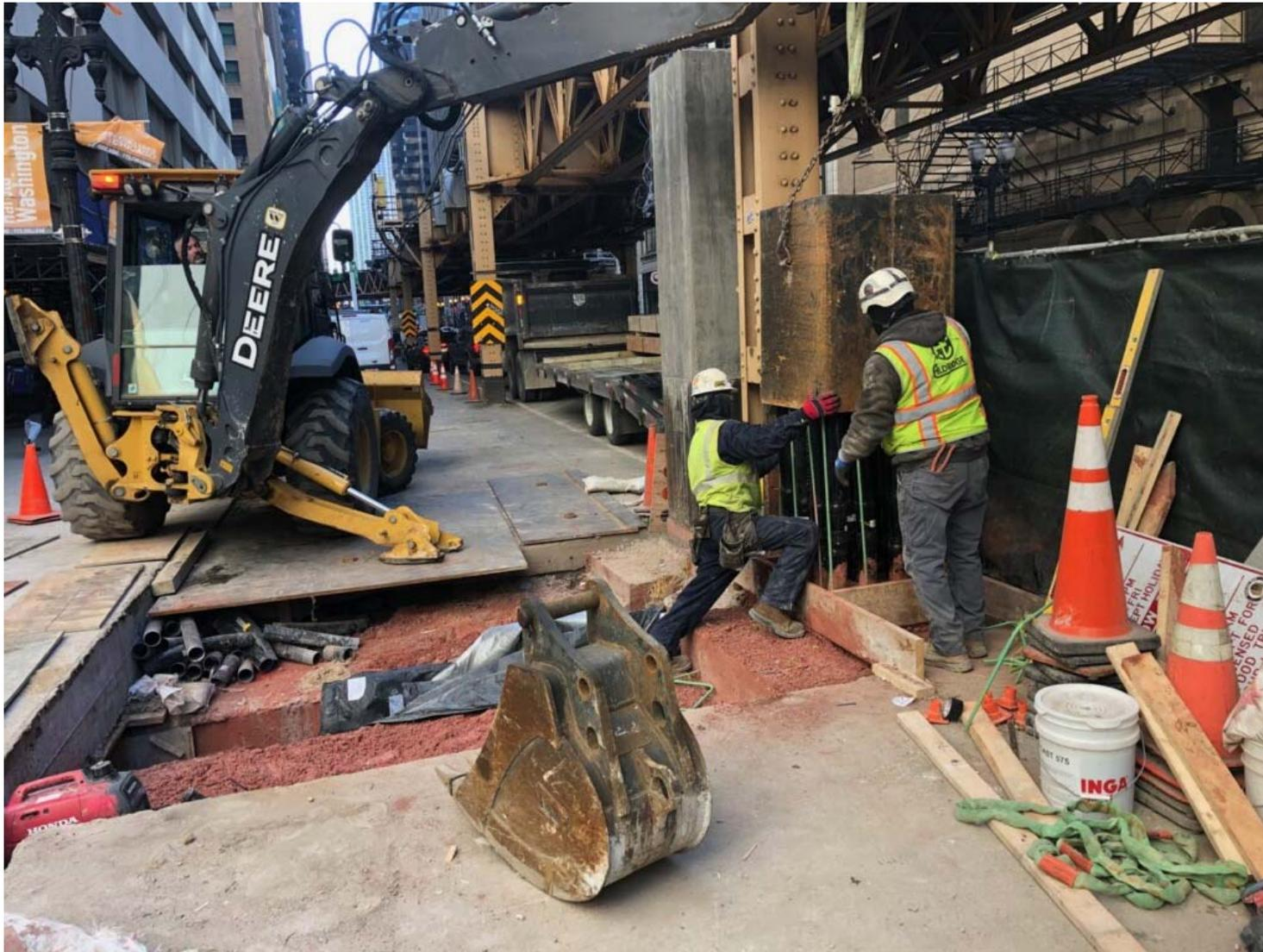
**Traction Power Ductbank Casing Installation at East Lake Substation**
