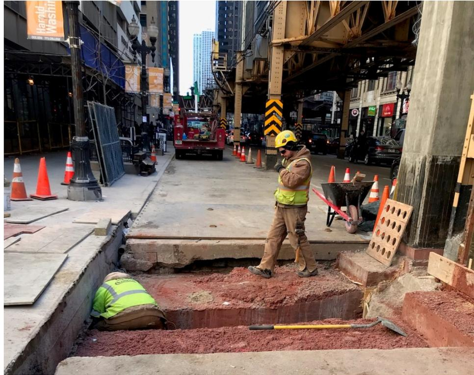
**Traction Power Ductbank Installation at East Lake Substation**
