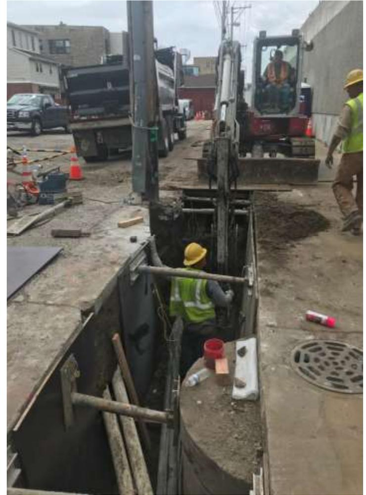
Water main installation by CDWM-Water on Sheffield (left) and ComEd trench excavation and shoring in east alley south of Lawrence (right)
