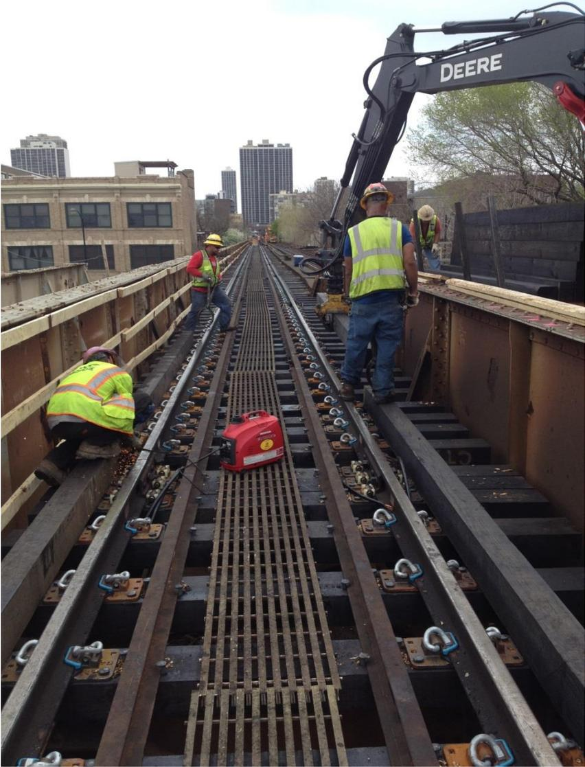
**Contractor Installing Timber Guard with New Track**
