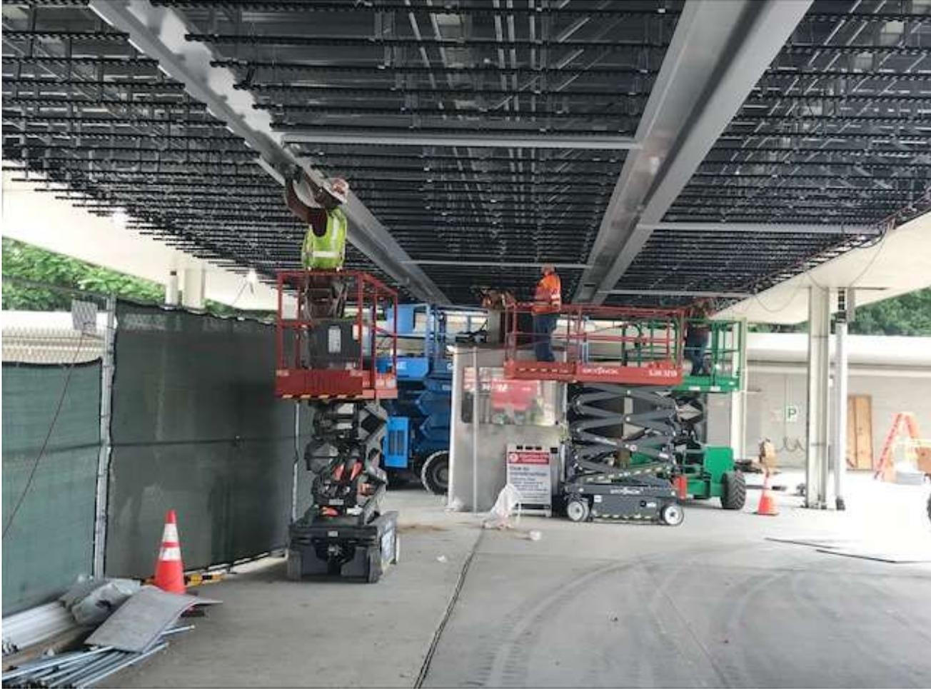
**Installation of Ceiling System at Jefferson Park Bus Terminal Walkway**
