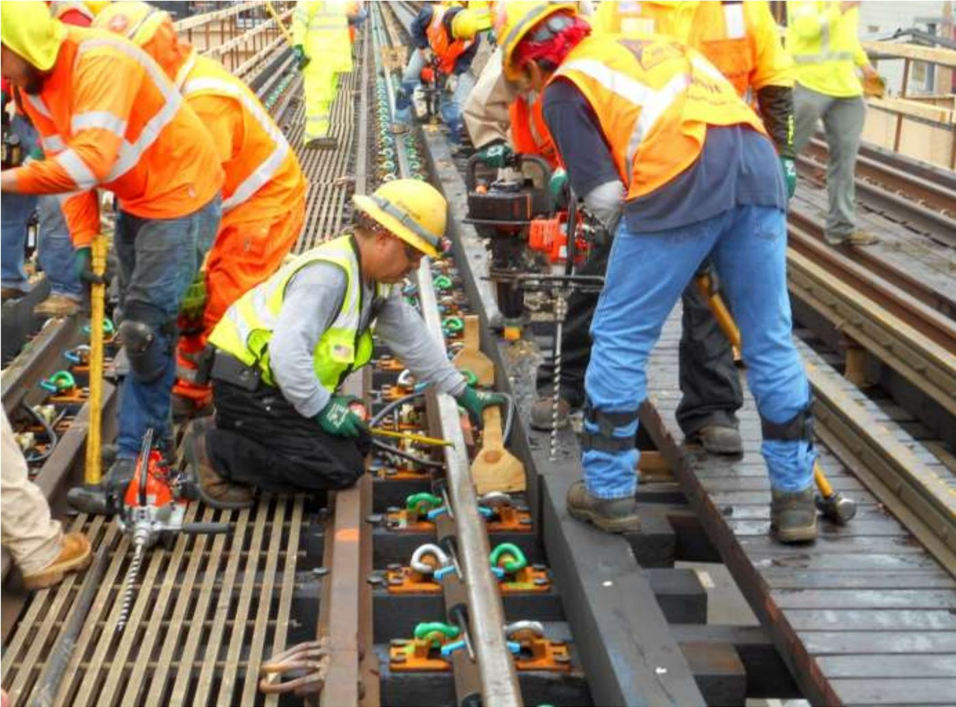
**Installing Track and Timber Guard**
