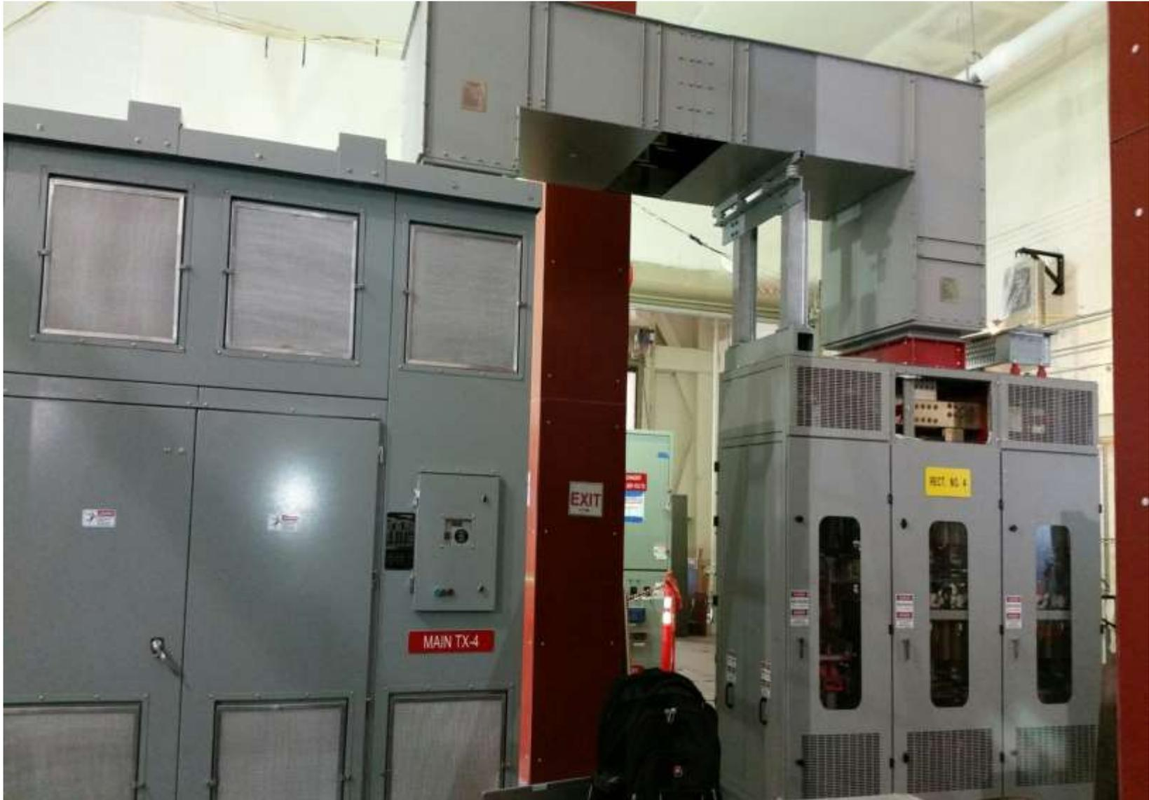
**Completed Installation of Lineup 4 Bus Duct**
