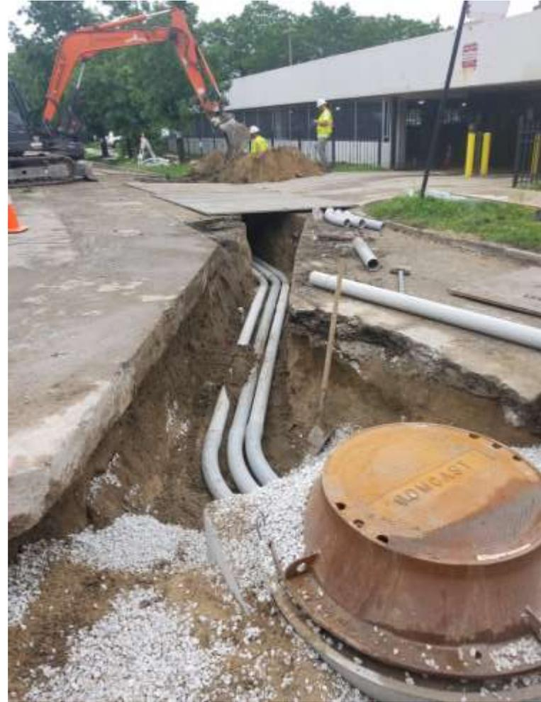
**Encased joint ductbank in east alley south of Lawrence (left) and installed conduits on Ainslie (right)**
