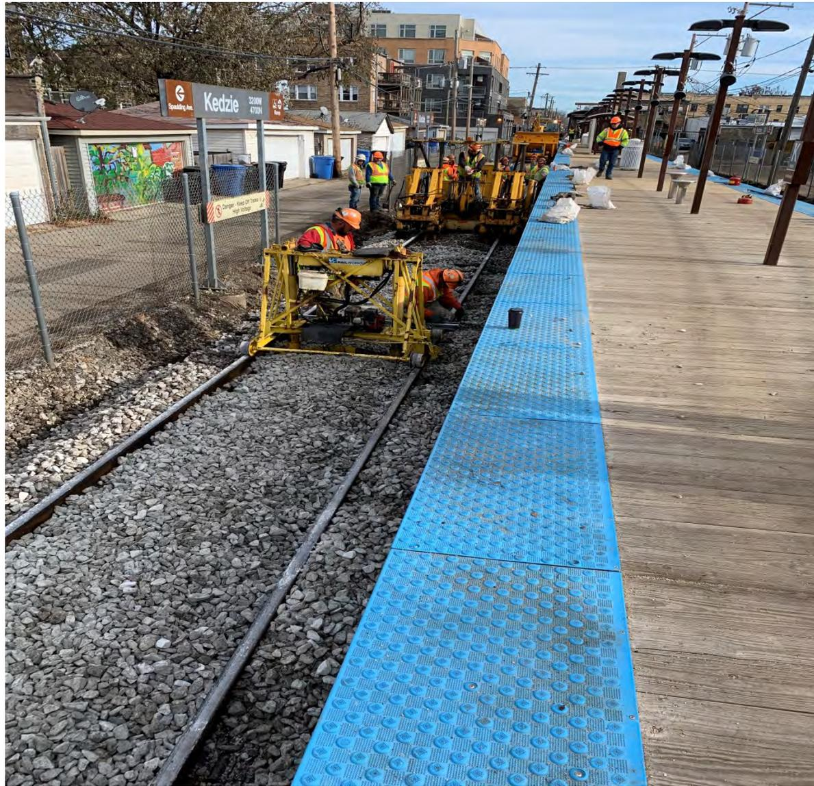
**Installation of Running Rail and Tamping**
