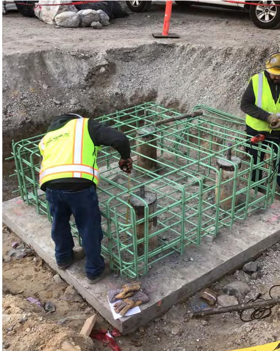
**Red-Purple Bypass – Placing Rebar Cage for Micropile Cap**
