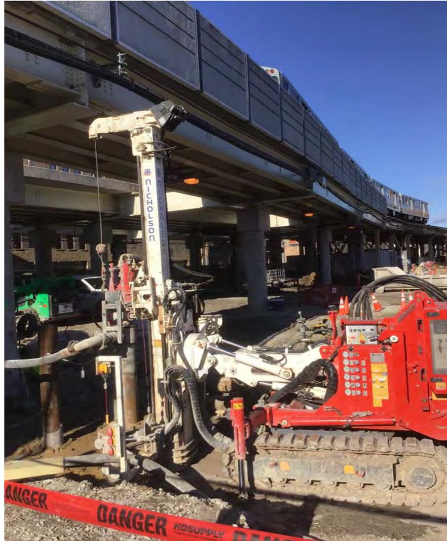
**Red-Purple Bypass – Installing Micropiles**
