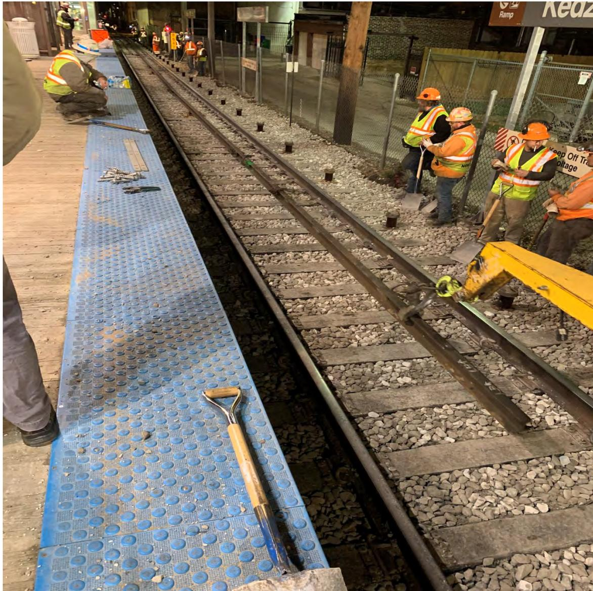
**Installing Auxiliary Negative Return Rail at Kedzie**
