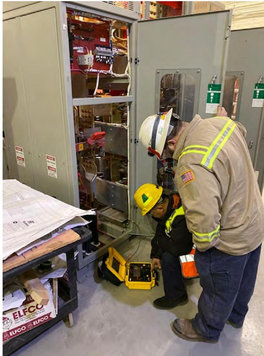
**Testing Rectifier at East Lake Substation**
