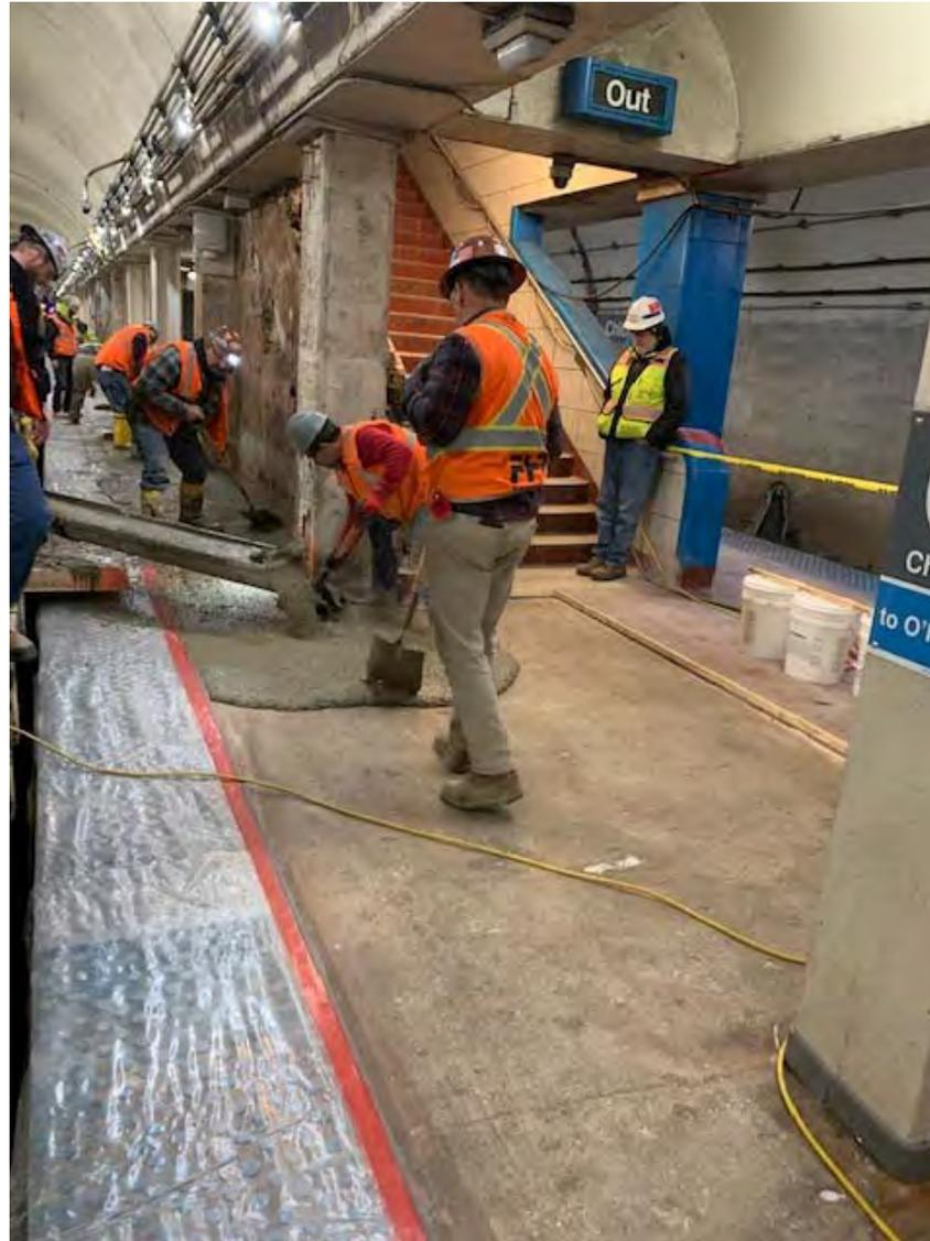
**Installation of New Platform Topping at Chicago Station**
