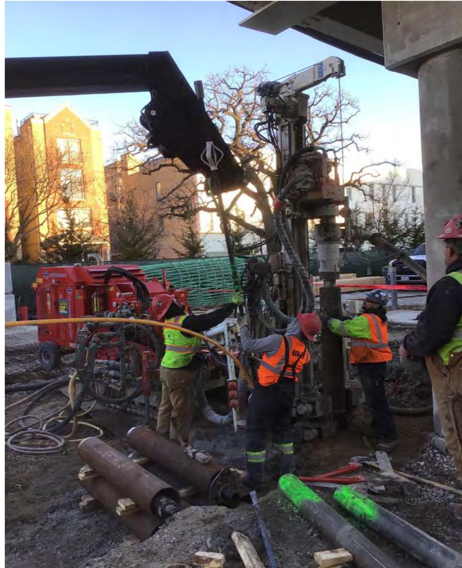
**Red-Purple Bypass – Installing Micropiles**
