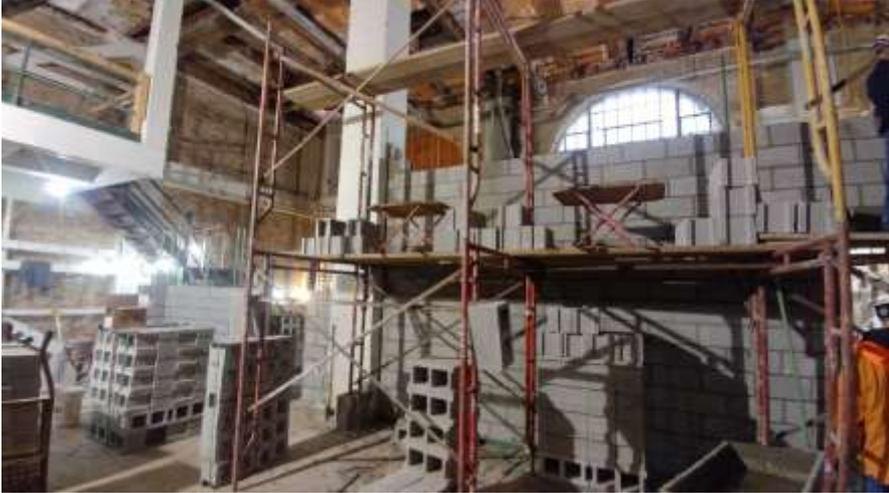
Interior CMU Wall Installation at East Lake Substation
