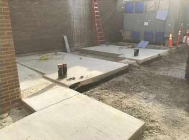
Concrete Transformer Pads Poured at Milwaukee Substation
