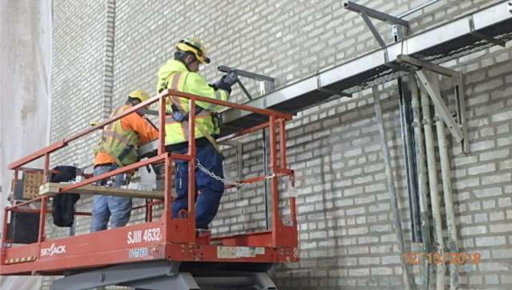
Installation of Bracket Supports for Cable Trays and Conduit
