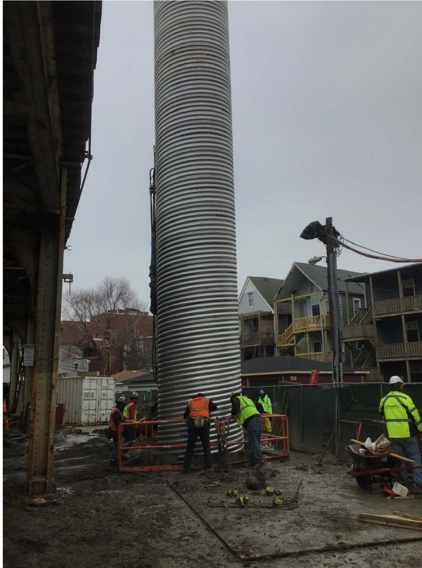
**Red-Purple Bypass: Installing Permanent Liner**
