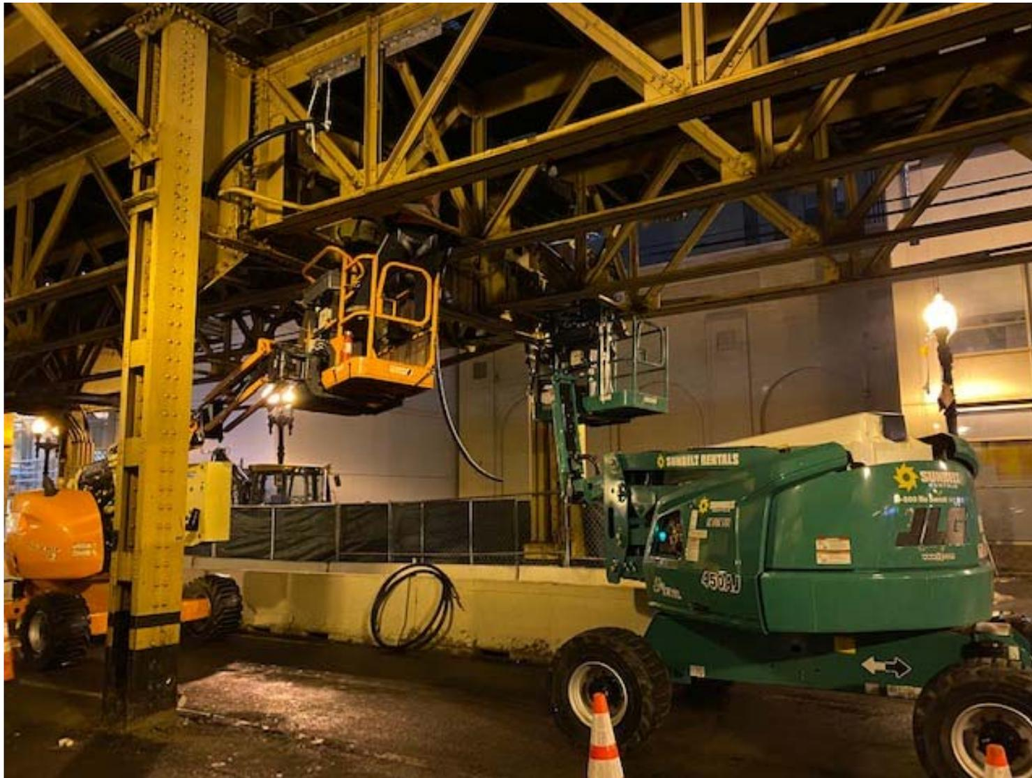
**Traction Power Cable Installation at East Lake Substation**
