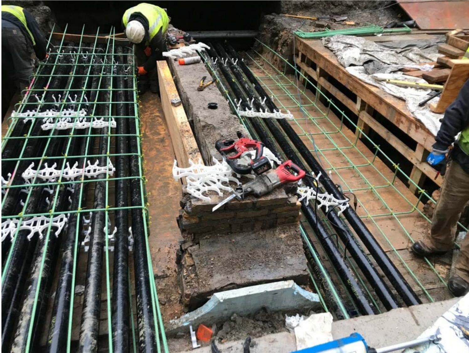
**Traction Power Ductbank Installation at East Lake Substation**
