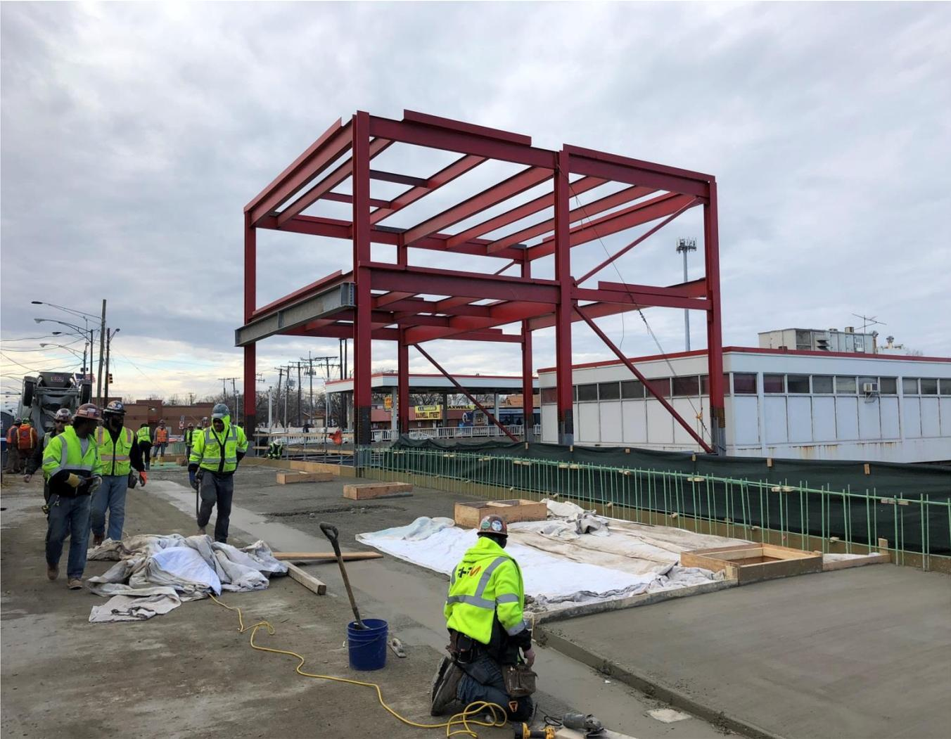
North Terminal: Bridge Extension Concrete Pour and Building Steel
