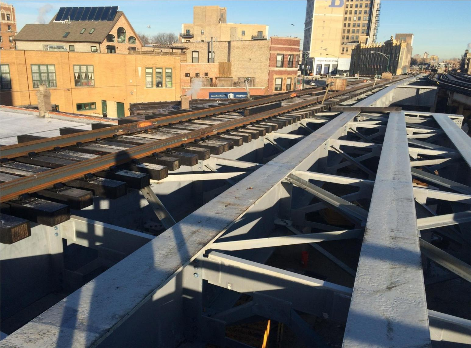
**New open deck track 1 rail and ties installation**
