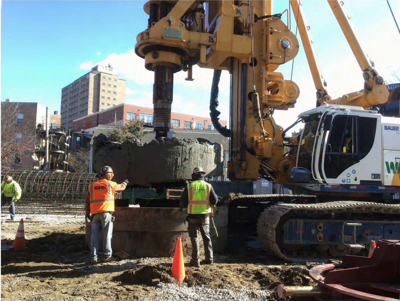
**Red-Purple Bypass – Drilling drilled shaft**
