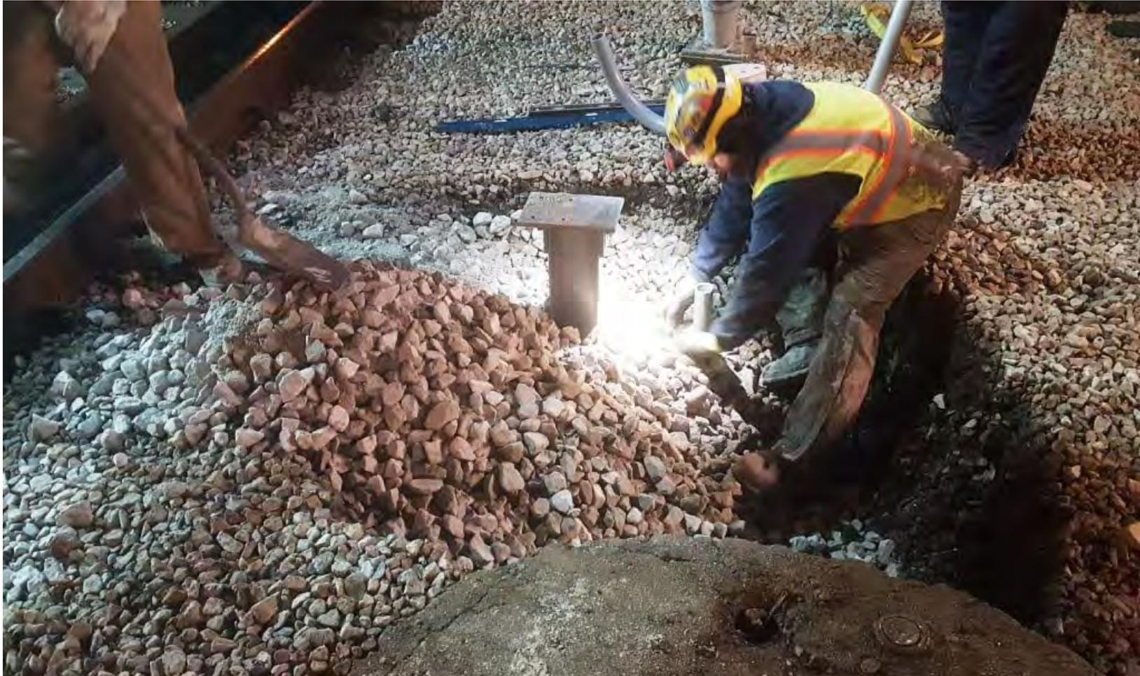
**Installation of I-Bond Foundations**
