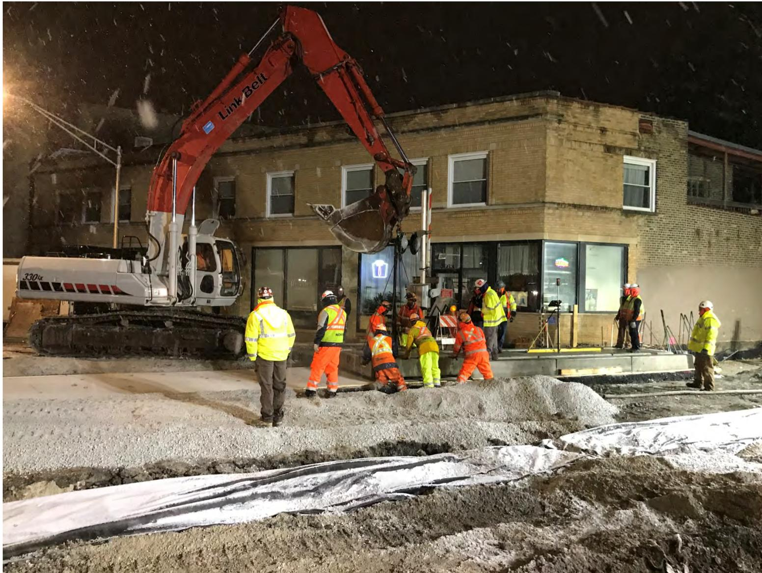
**Installation of Precast Concrete Crossing Panels**
