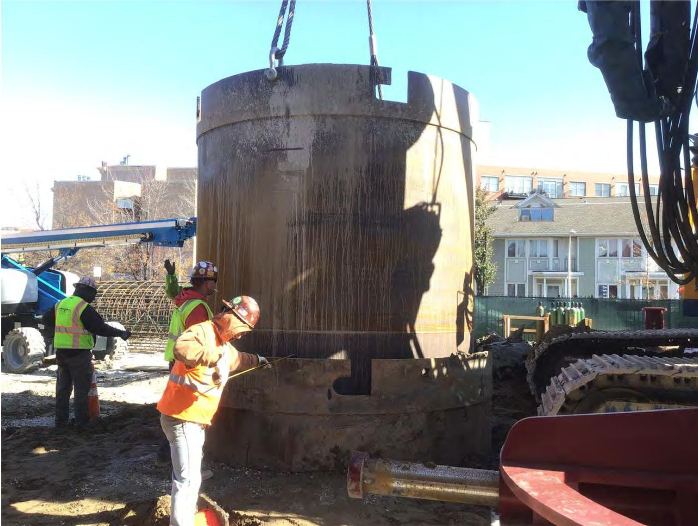
**Red-Purple Bypass – Installing temp steel casing in drilled shaft**
