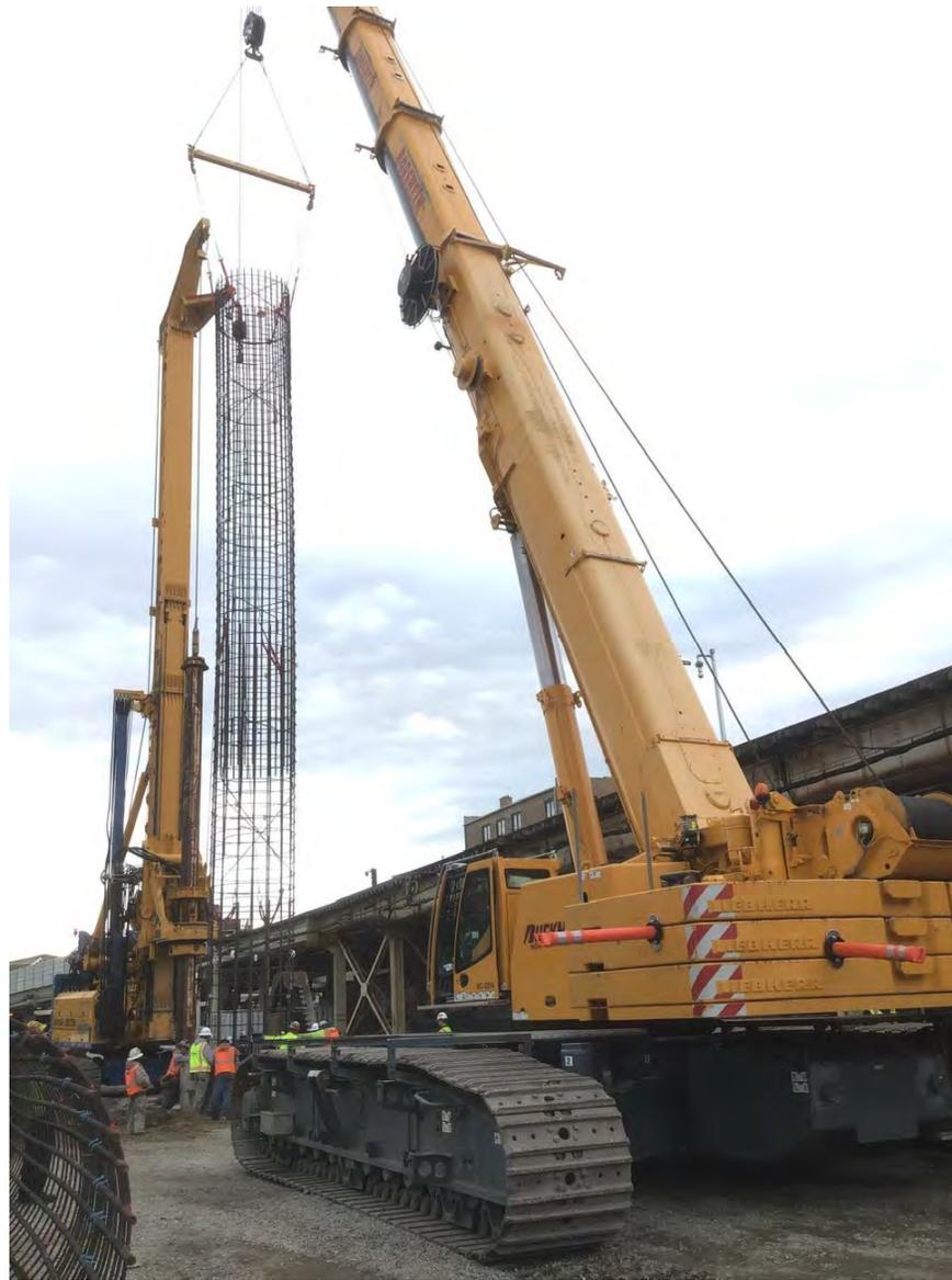
**Red-Purple Bypass – Placing rebar cage for drilled shaft**
