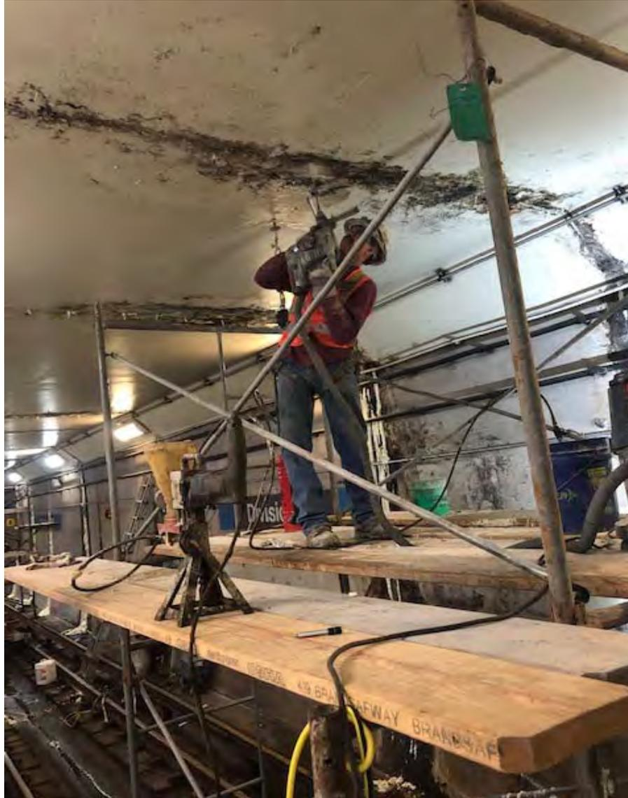
**Grout Injection for Water Mitigation at Division Station**
