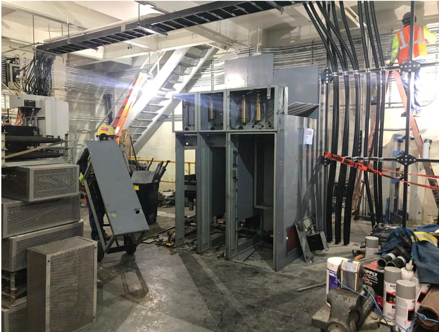
**DC Switchgear Demolition at East Lake Substation**
