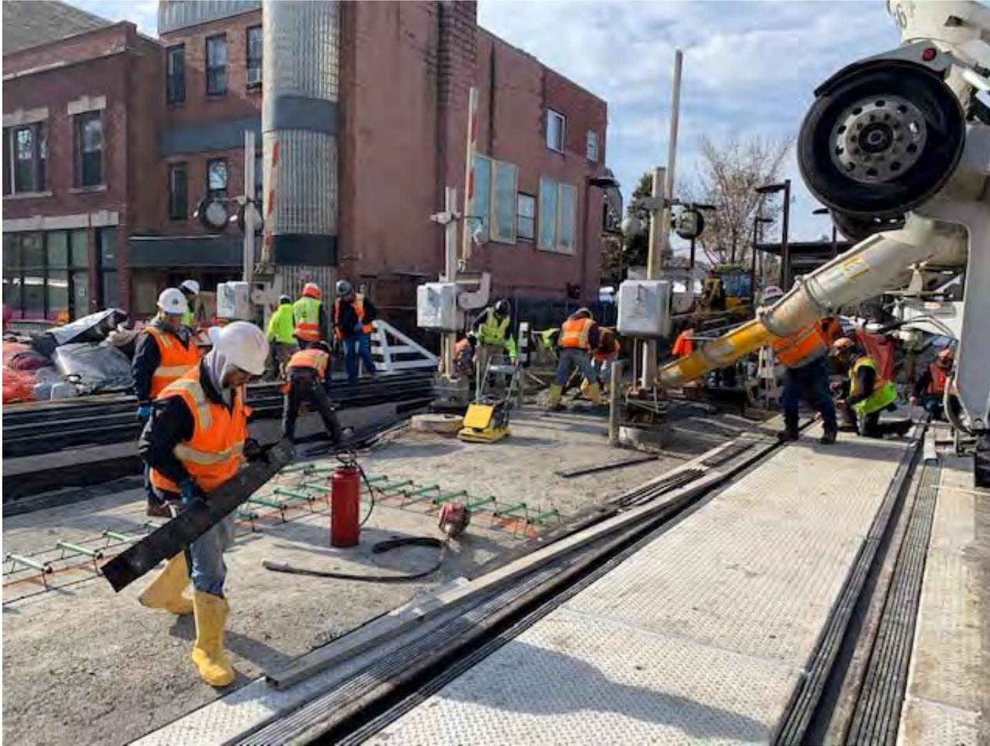
**Installation of Rail Crossing Concrete and Sidewalk**
