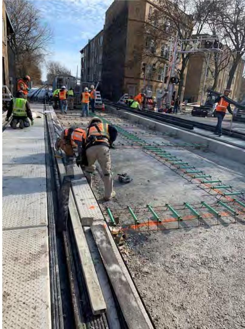
**Installation of Reinforcement for Concrete Crossing**
