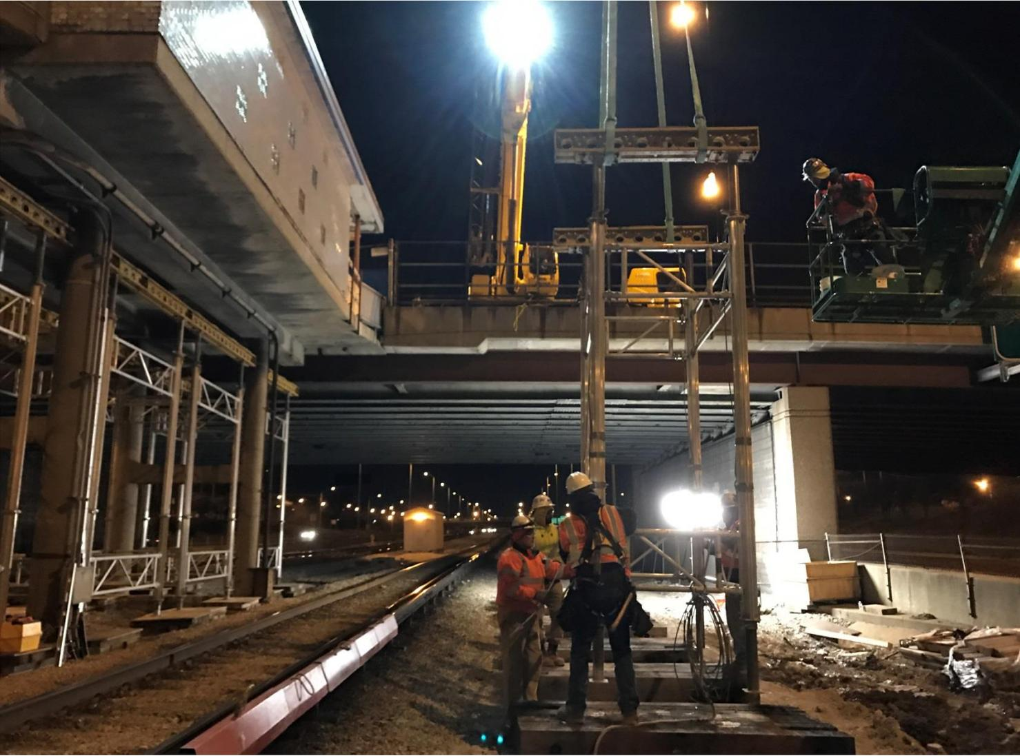
**Damen Stationhouse temporary work platform tower erection**
