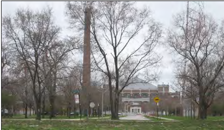
Figure 4: Block Park with the Roseland Pumping Station in the Background (facing south)
