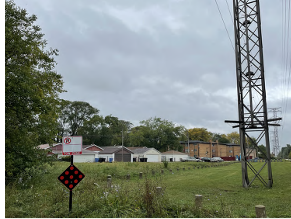
VIEW FROM WALLACE STREET FACING NORTH
