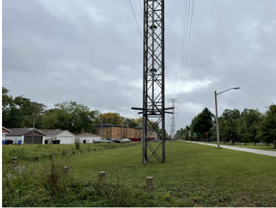
VIEW FROM WALLACE STREET FACING NORTH
