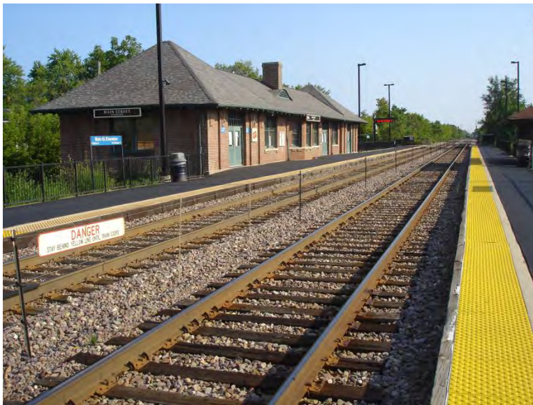
Figure 5-3: Intertrack Fencing at a Metra Station
