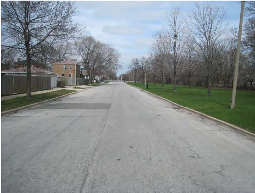
Figure 4-6: Fernwood Parkway at 100th Street and Eggleston Avenue (facing north)
