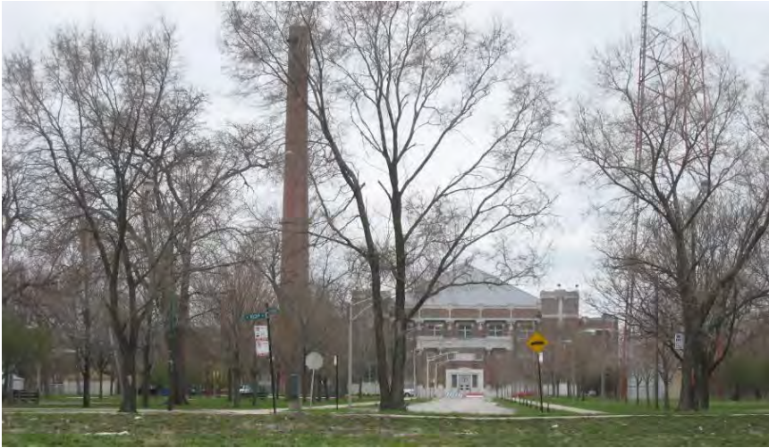
Figure 4-8: Block Park Facing South with the Roseland Pumping Station in the Background (facing south)
