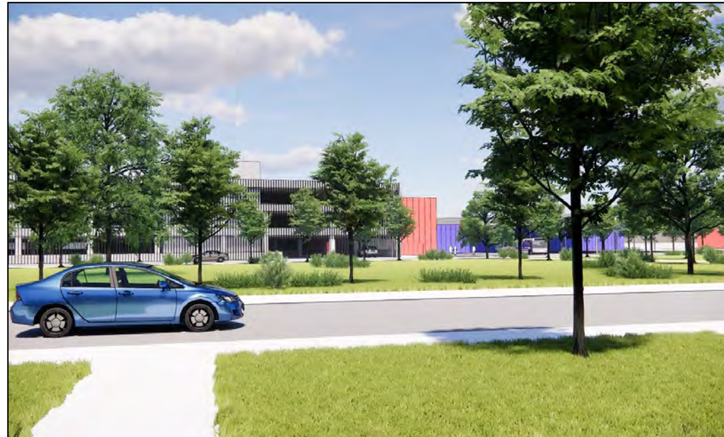
Photo Simulation of the 130th Street Station, Facing East from the Eastern Edge of the Altgeld Gardens Neighborhood
