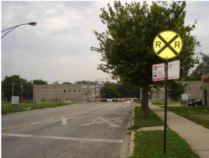
Figure 4-3: 111th Street at the Union Pacific Railroad tracks, looking west
