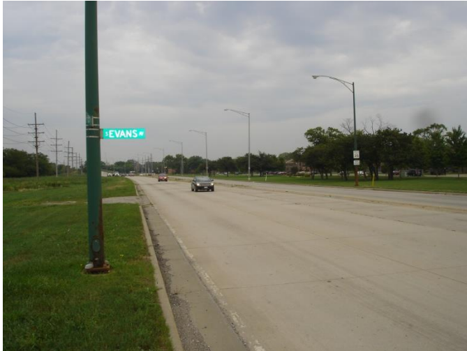
Figure 4-4: 130th Street at Evans Avenue, looking east
