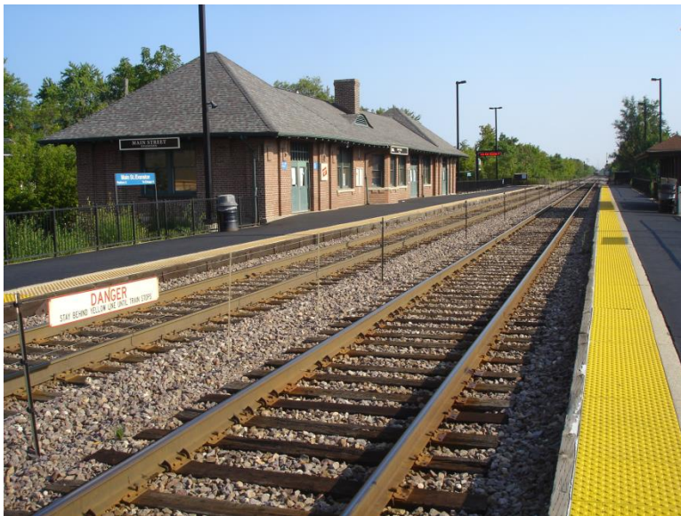
Figure 5-3: Intertrack Fencing at a Metra Station
