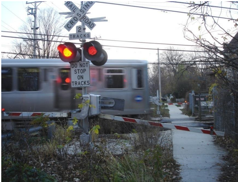
Figure 5-2: Pedestrian Crossing Gates at Isabella Street on Chicago Transit Authority Purple Line
