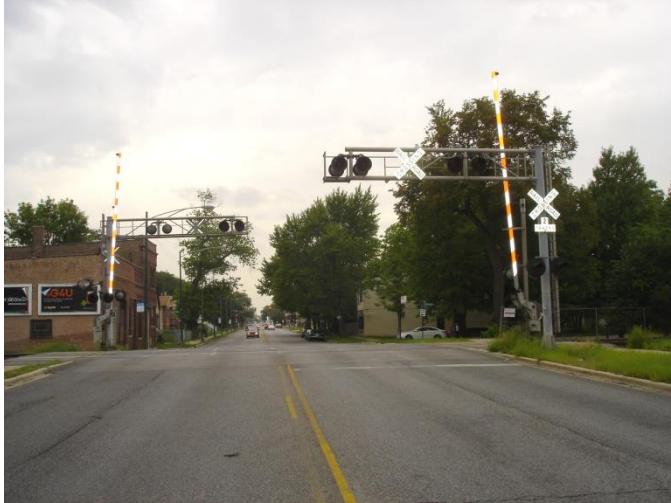
Figure 4-2: 103rd Street at the Union Pacific Railroad tracks, looking west
