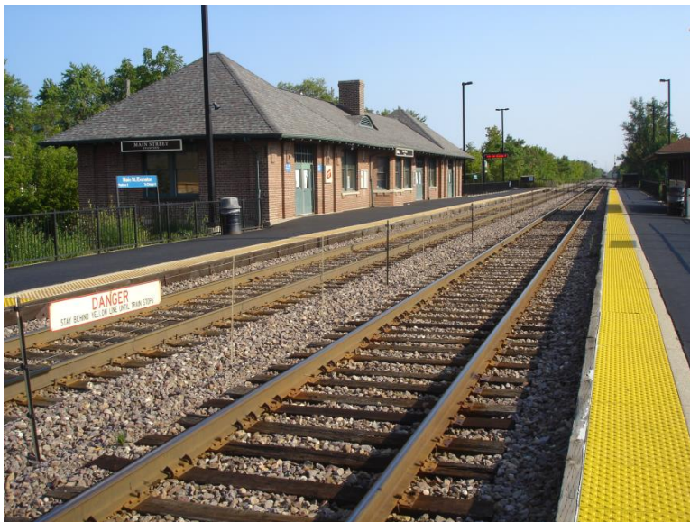
Figure 5-3: Intertrack Fencing at a Metra Station
